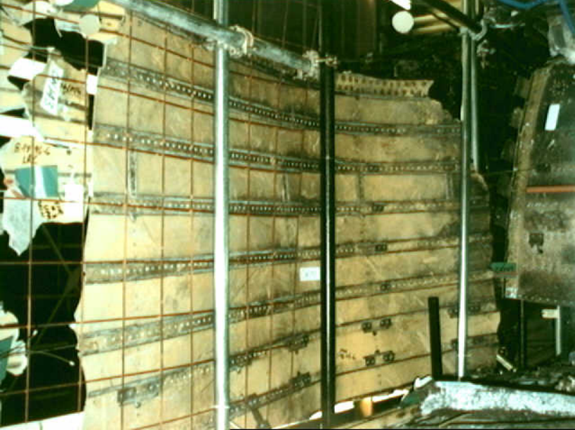
Structures 7 - CW-135 Photo 1
