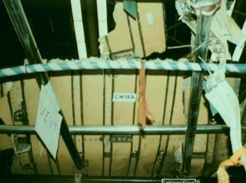
Structures 7 - CW-122 Photo 1
