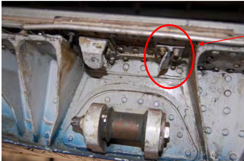
Aft, frame 55A
