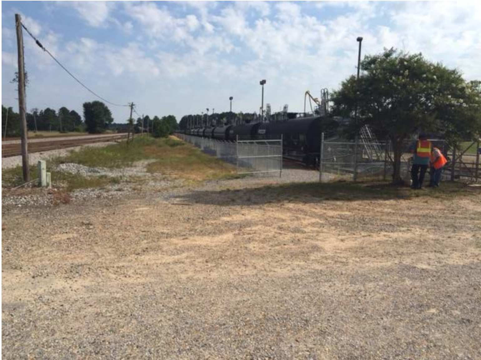
Photo looking at gate at south end (end of tracks) in plant.
