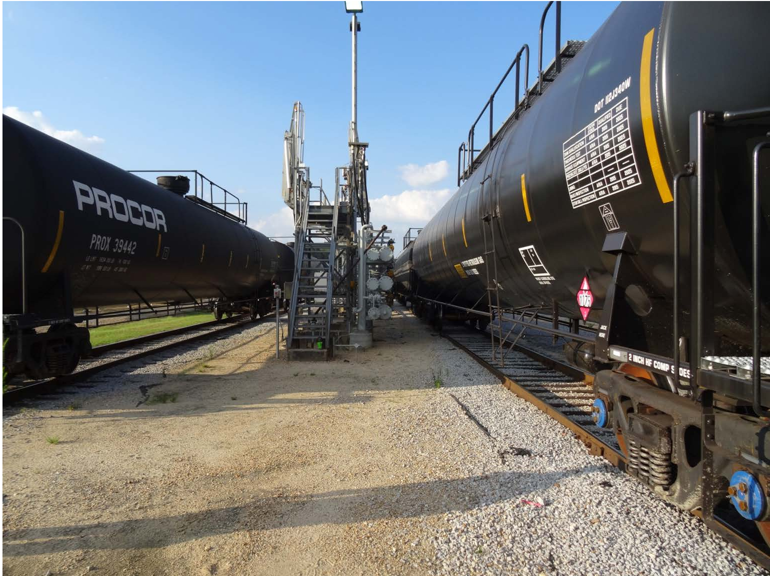
Photo facing south, showing two tracks separated by pipe rack
