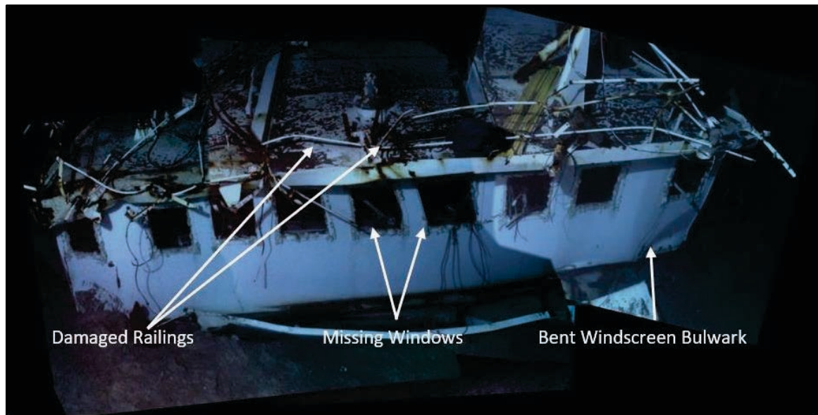
Figure 27. Bridge and bridge deck, looking aft. (Photomosaic image from mission 2)
