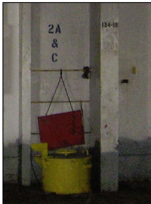
Figure 58. Second deck scuttle to hold 2A, similar to hold 3 scuttle. (Photo by Herbert Engineering)
