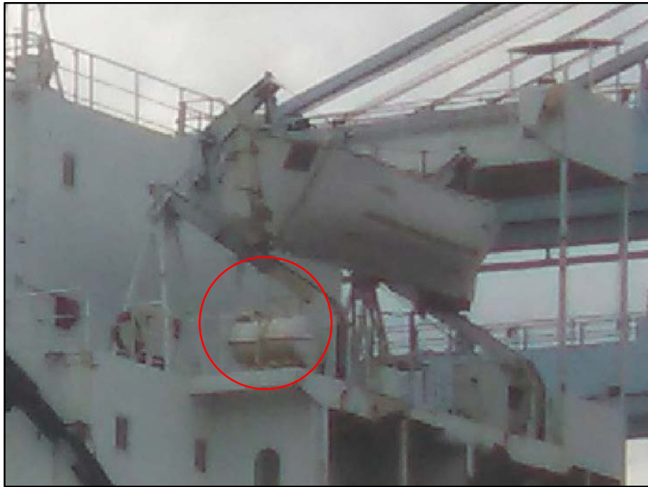
Figure 49. Location of liferaft stowed below El Faro's starboard lifeboat. (Photo by Maine Maritime Academy cadet, summer 2015)
