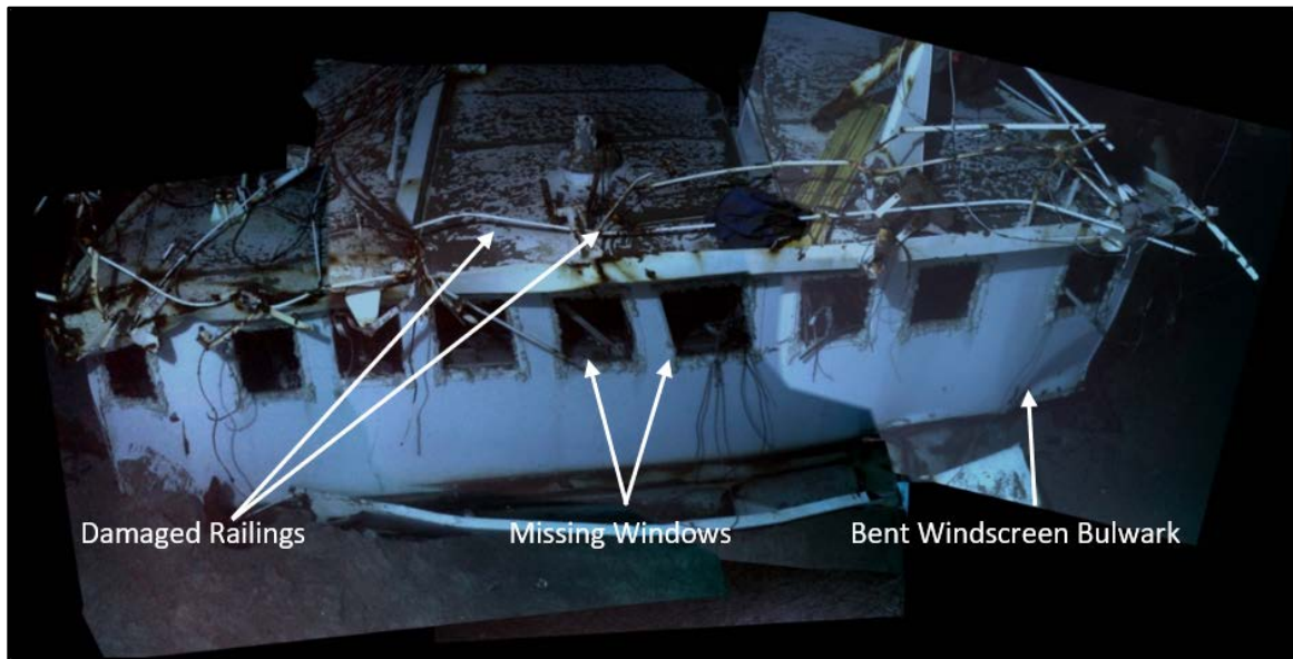
Figure 27. Bridge and bridge deck, looking aft. (Photomosaic image from mission 2)
