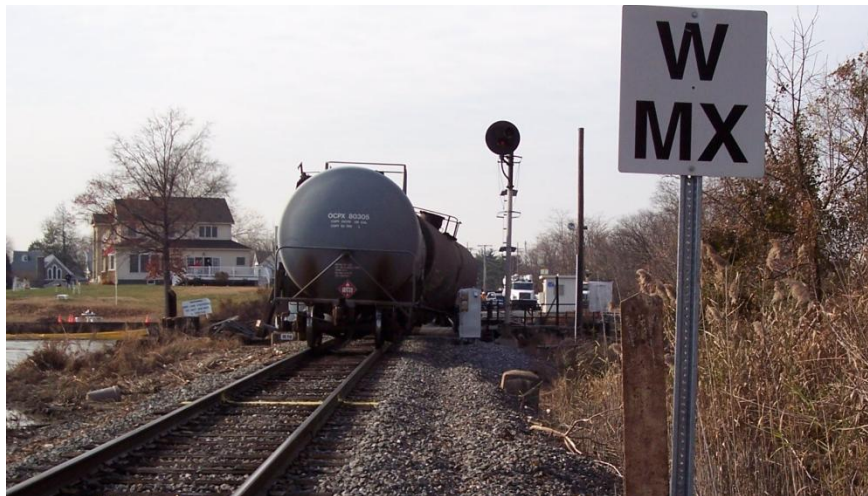
Figure 3. View of 1S Signal at Paulsboro Moveable Bridge
