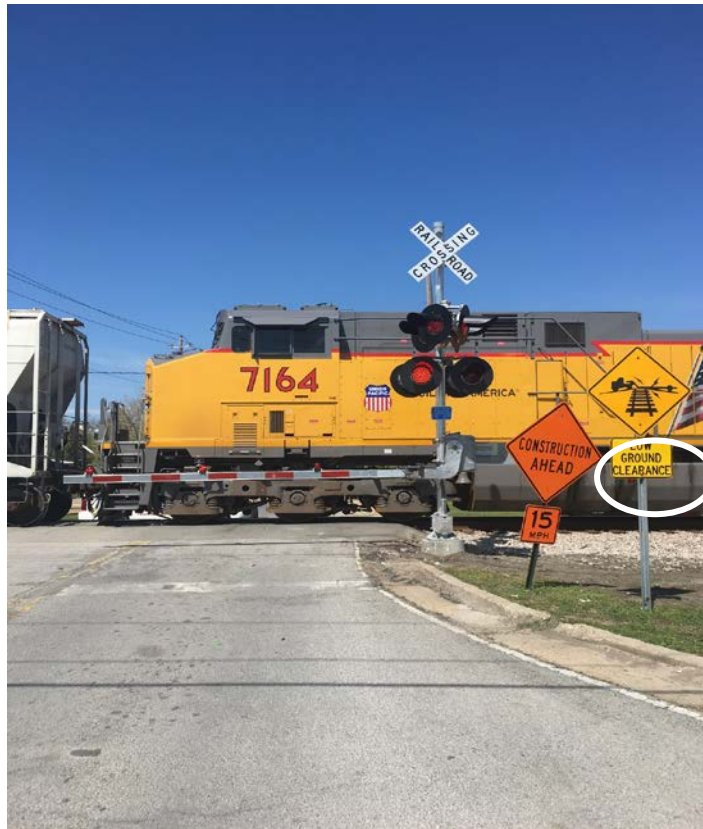
Figure 2. Photo of the repaired signal gate and flasher. White circle highlights low ground clearance sign.
