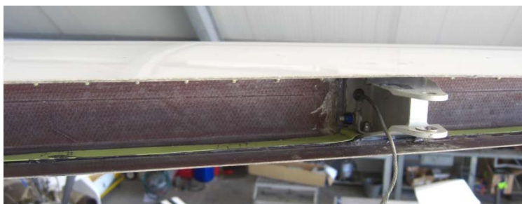
Fig.2 – Center Fitting with aluminum bonding strips installed
