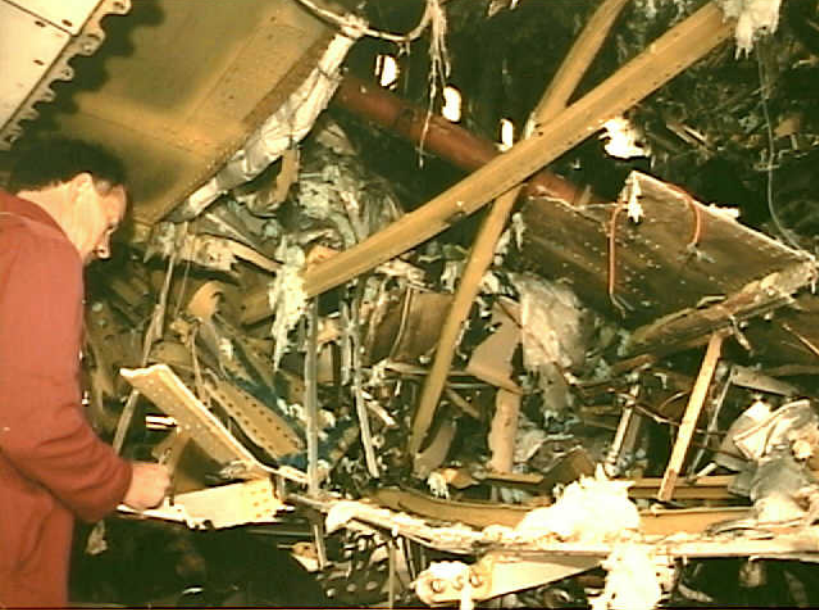
Sequencing Group 18 - Appendix B - Photo 7. Close-up view of the damage to wing center section.
