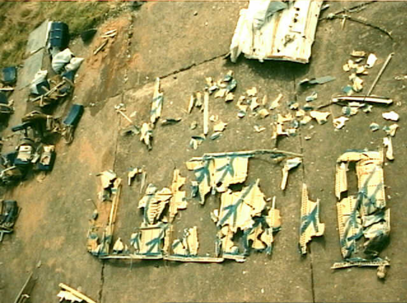
Sequencing Group 18 - Appendix B - Photo 11. View showing deformation & damage to SWB#3.
