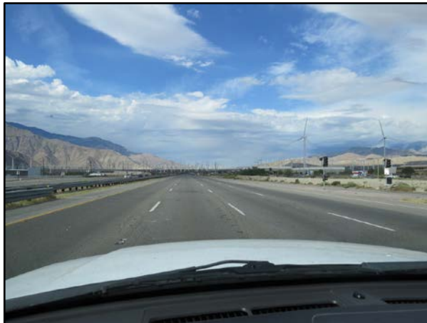
Figure 2. View of Interstate 10 westbound (looking west), approximately 2,505 feet east of the MCI.
