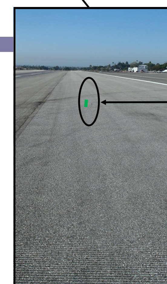
(A) First indication of landing gear ground contact. Light black transfer mark about 64-inches-long, consisting of 3 treads from the right main landing gear tire.
