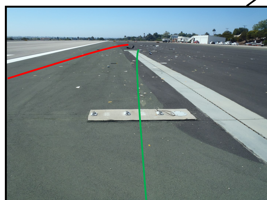
(D) Five tread marks from the right main landing gear tire beyond the remnants of a taxiway sign. Light scuffing of tarmac surface created by left main landing gear tire
