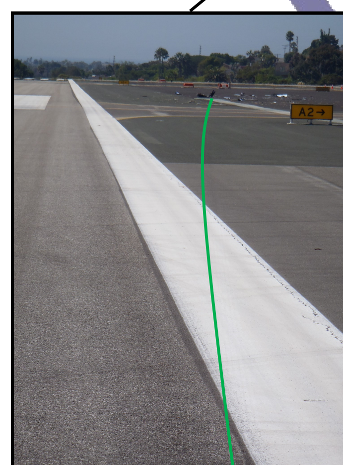
Light scuffing on the runway border displaying 5 treads of the right main landing gear tire.
