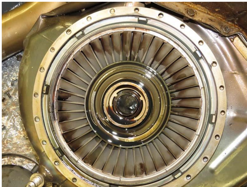
Power Turbine Rotor in Position inside exhaust Collector Support
