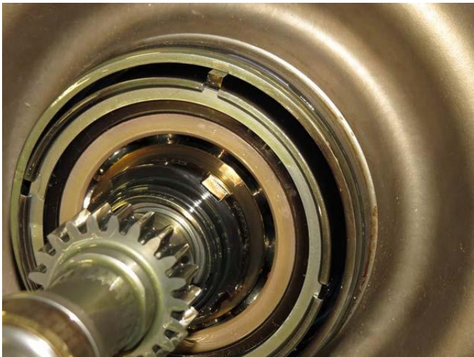
# 2 Bearing in Position
