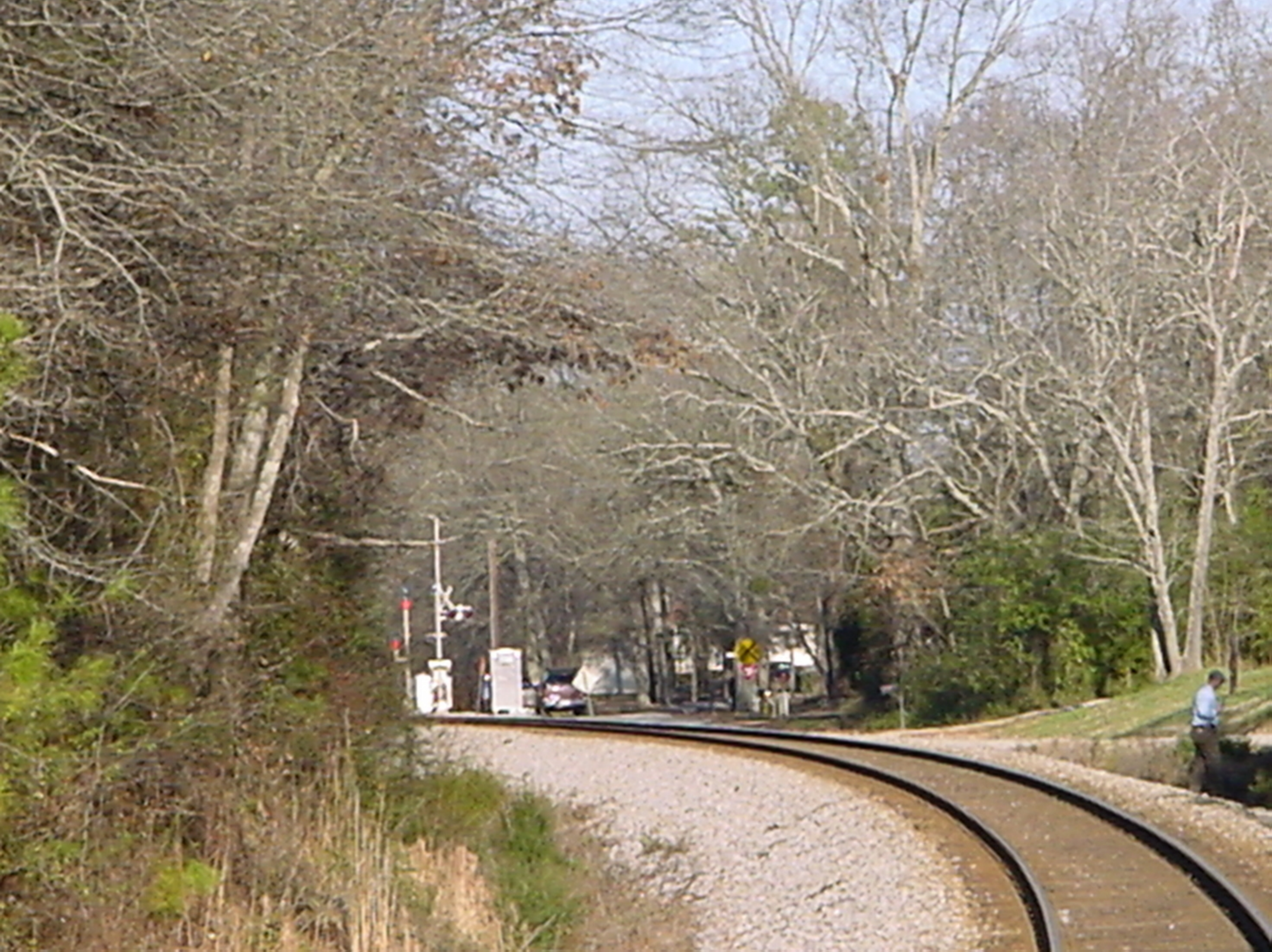
Riverside Signal No.760.4 Phantom Indication-Rule 309C Restricting Displayed (Double Red with number plate)Proceed at Restricted Speed
