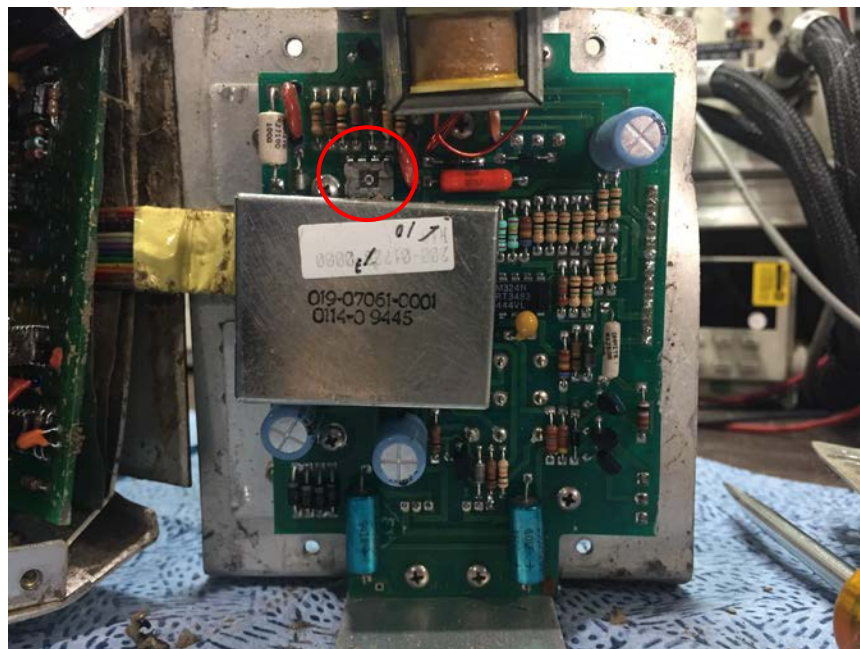
KC 295 Power Supply board – damaged part circled above (not testable)
