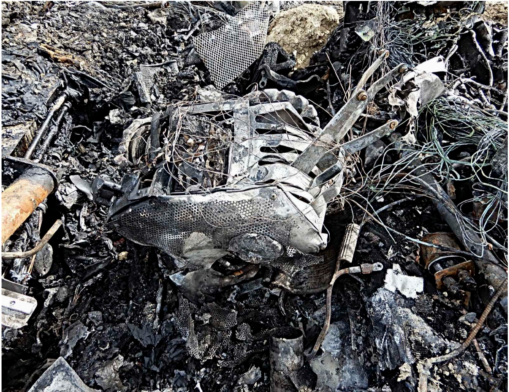
Photo 10 – The power quadrant.
