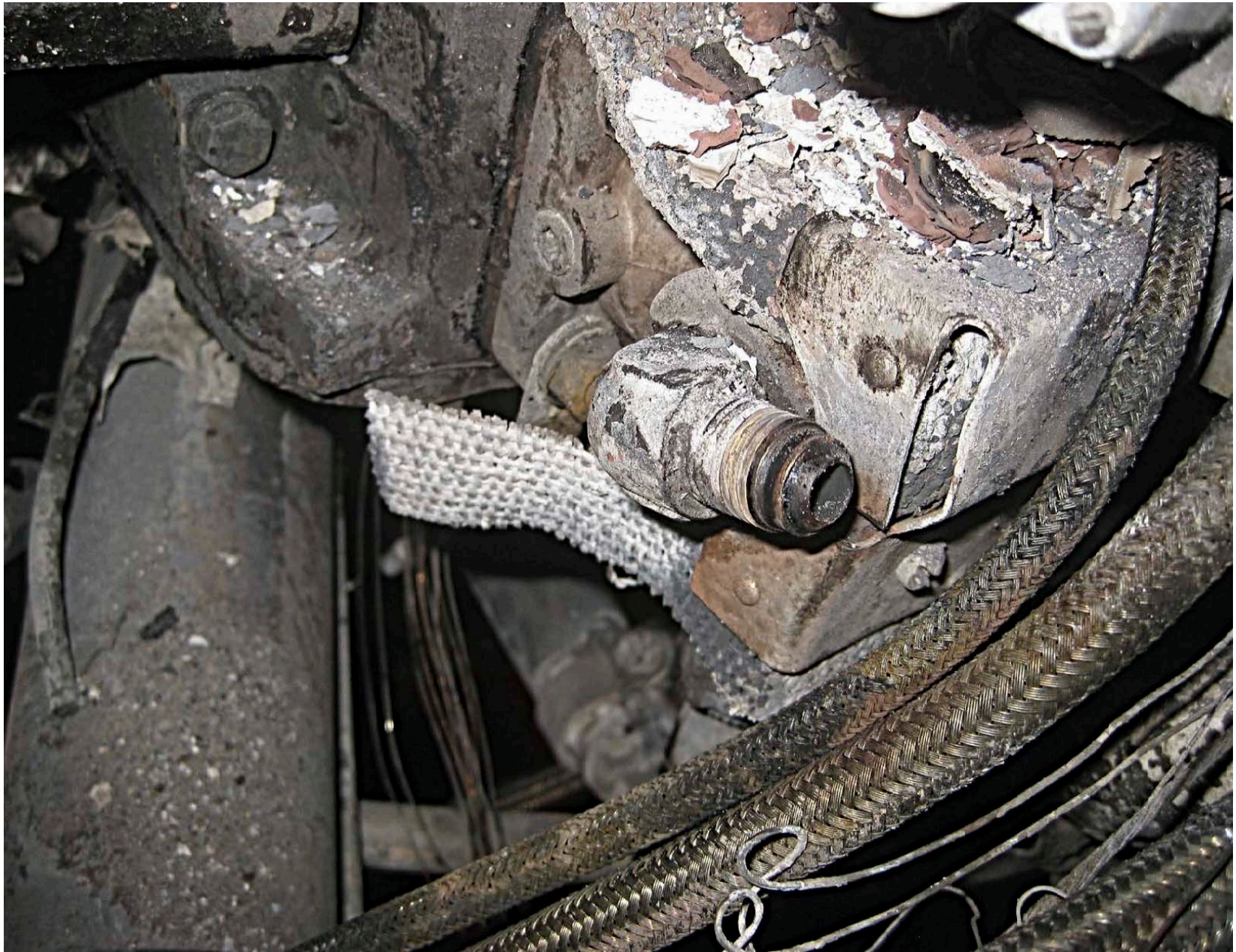
Photo 16 - Another view of the fuel pump discharge after line removal.
