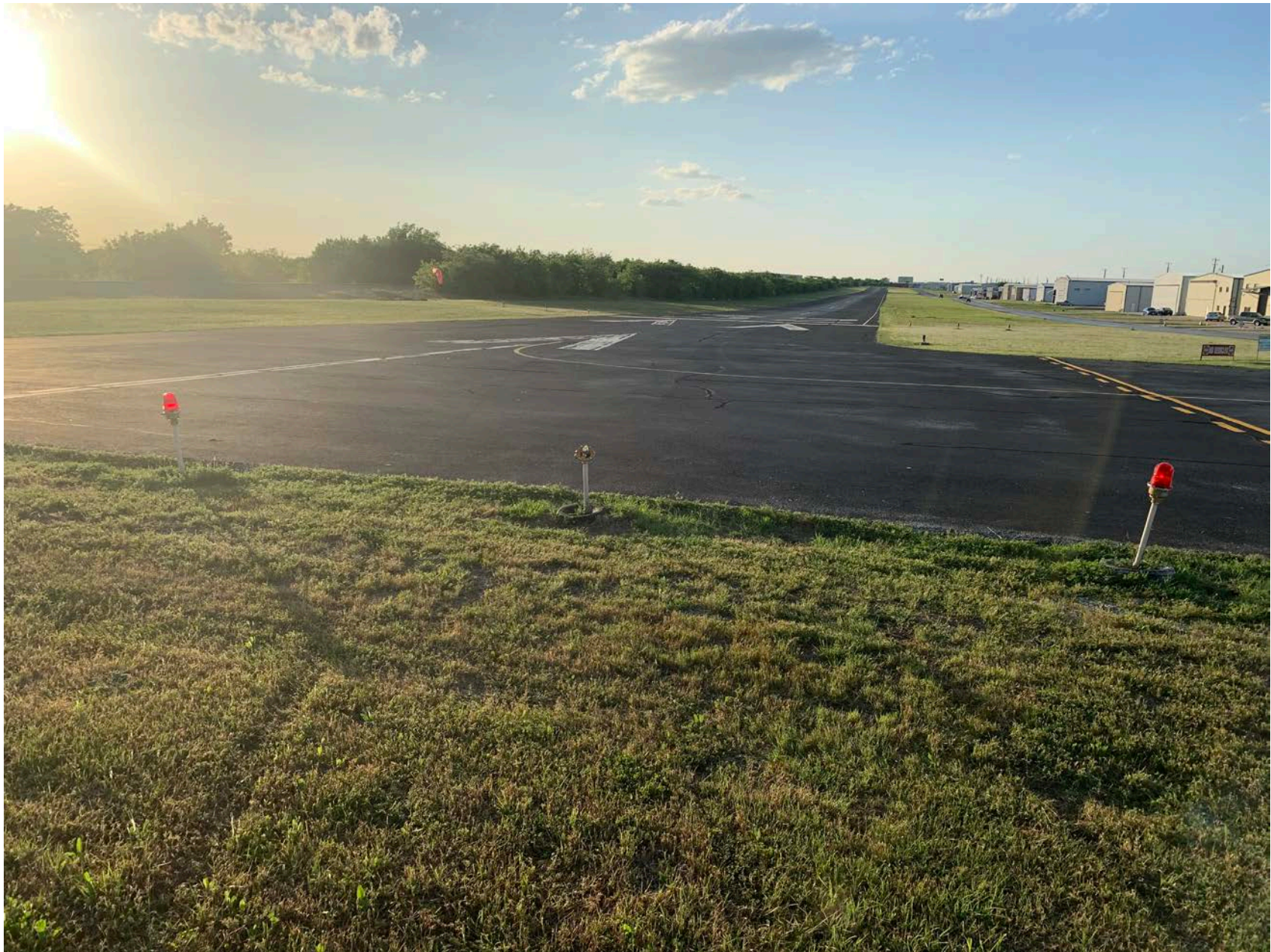
Photo 1 – View towards the departure end of runway 14. Note tire tracks and toppled airport lights (FAA photo)
