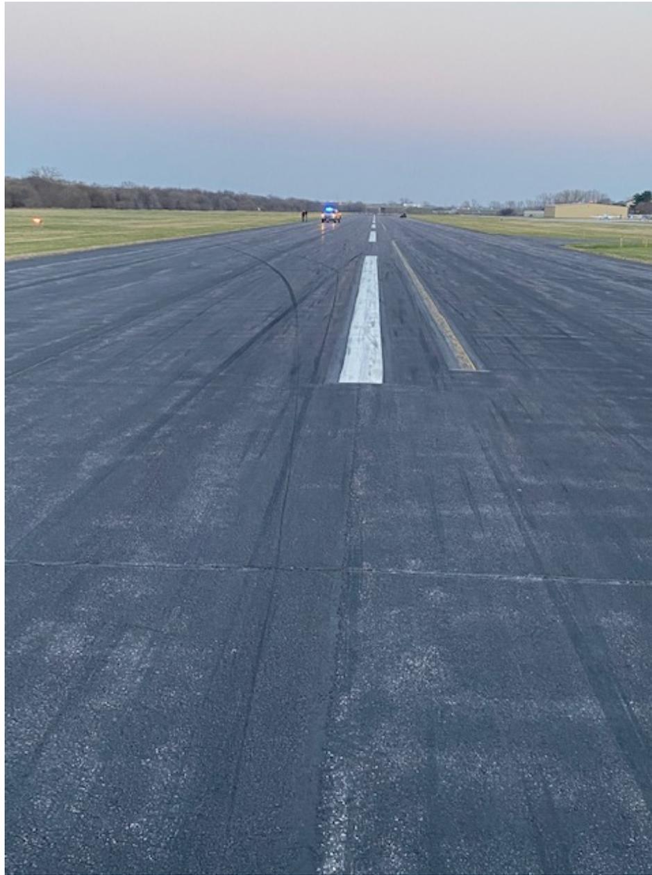
**Photo 1 – View to the southeast down runway 12. Note the skid mark angling off to the left (FAA photo)**
