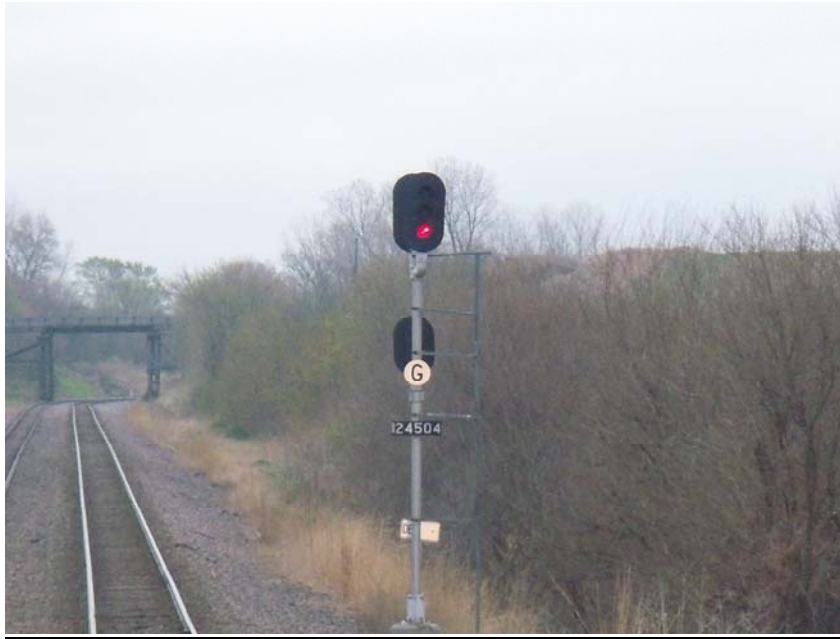
Figure 2. Intermediate Signal 24504 with Grade Marker.
