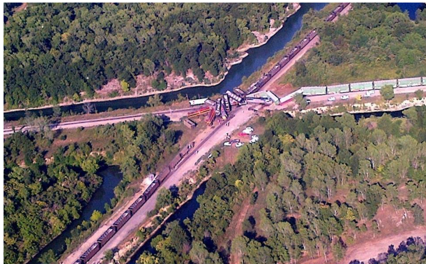
Figure 1. The accident site.
