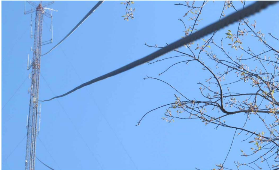
Guy wires on C side appear to be kinked and stretched
