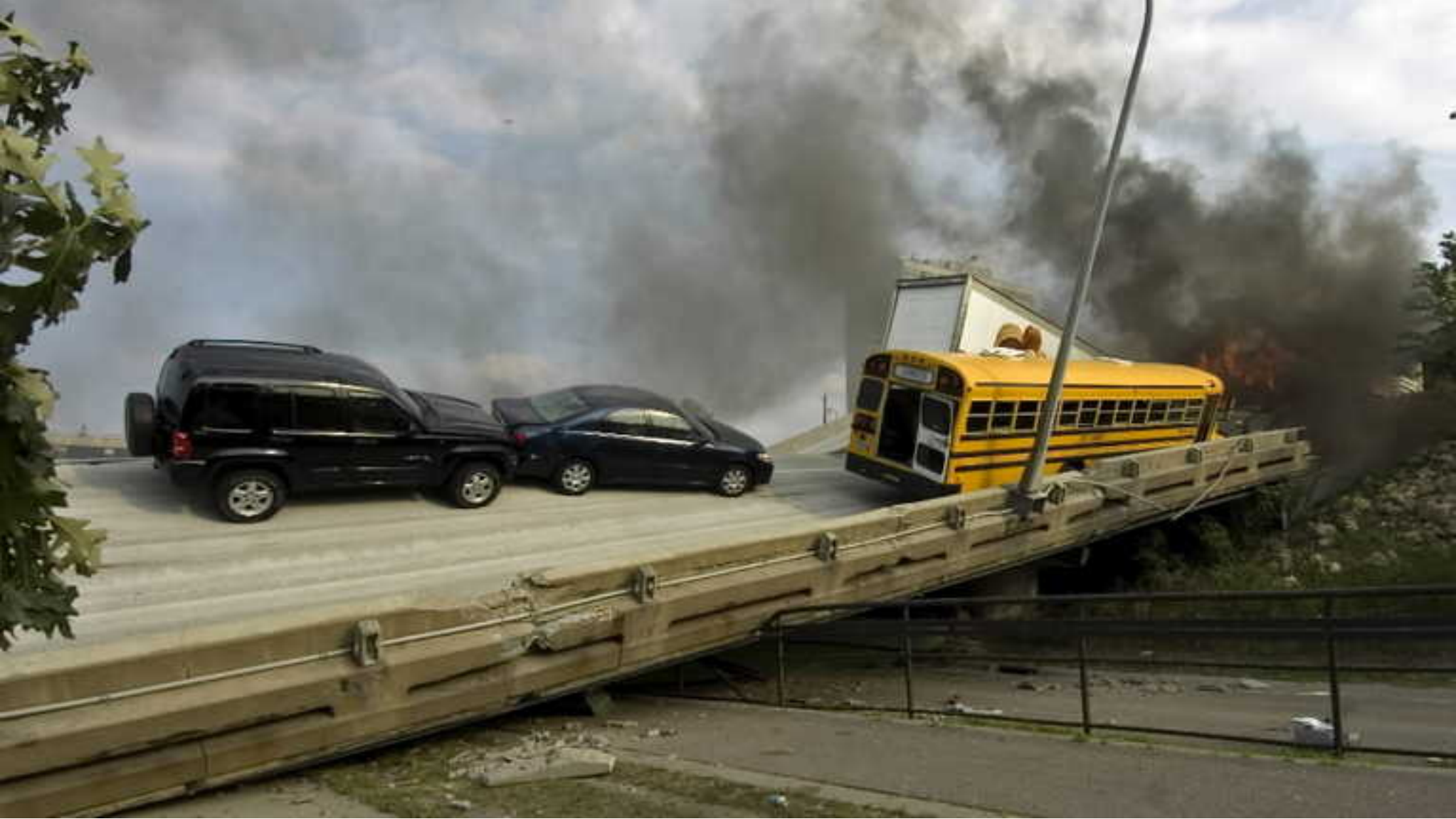
Presentation 07 - Photo of post-collapse vehicles
