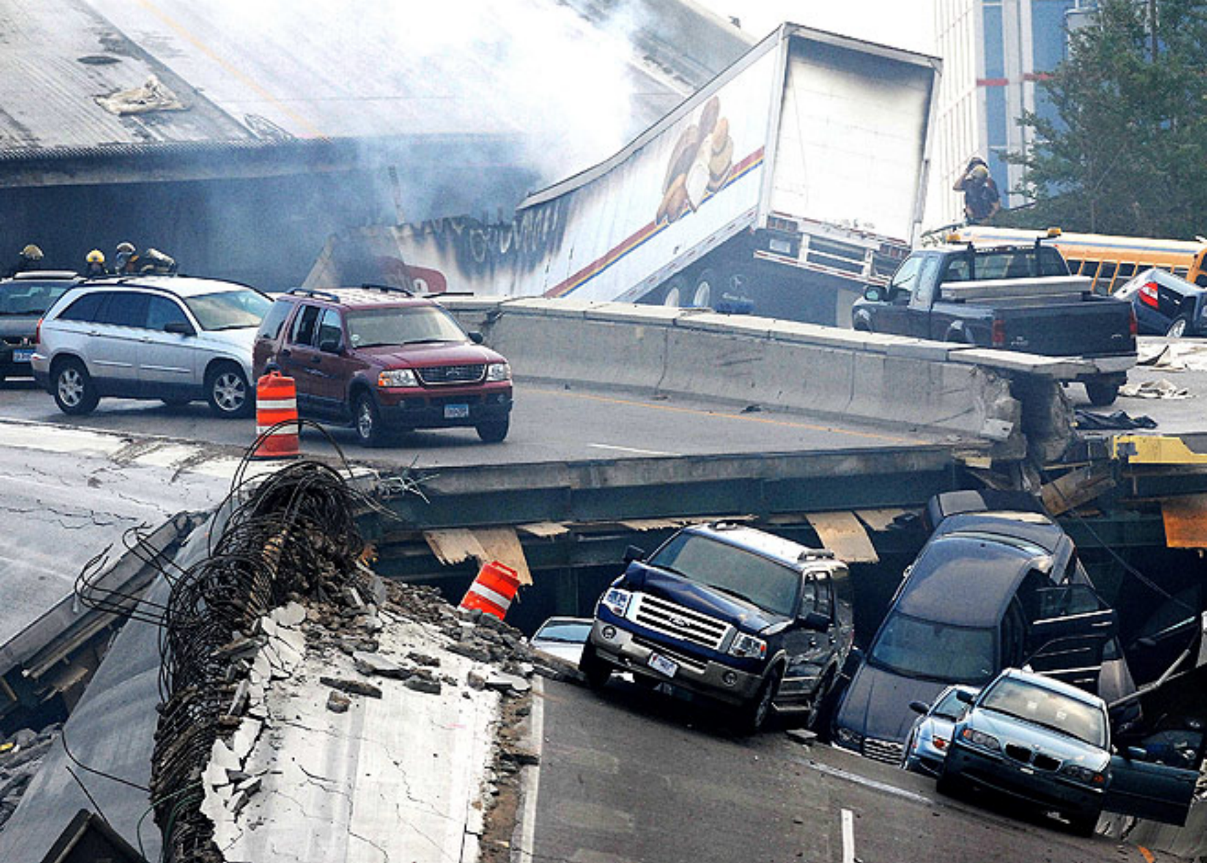
Presentation 06 - Photo of post-collapse vehicles
