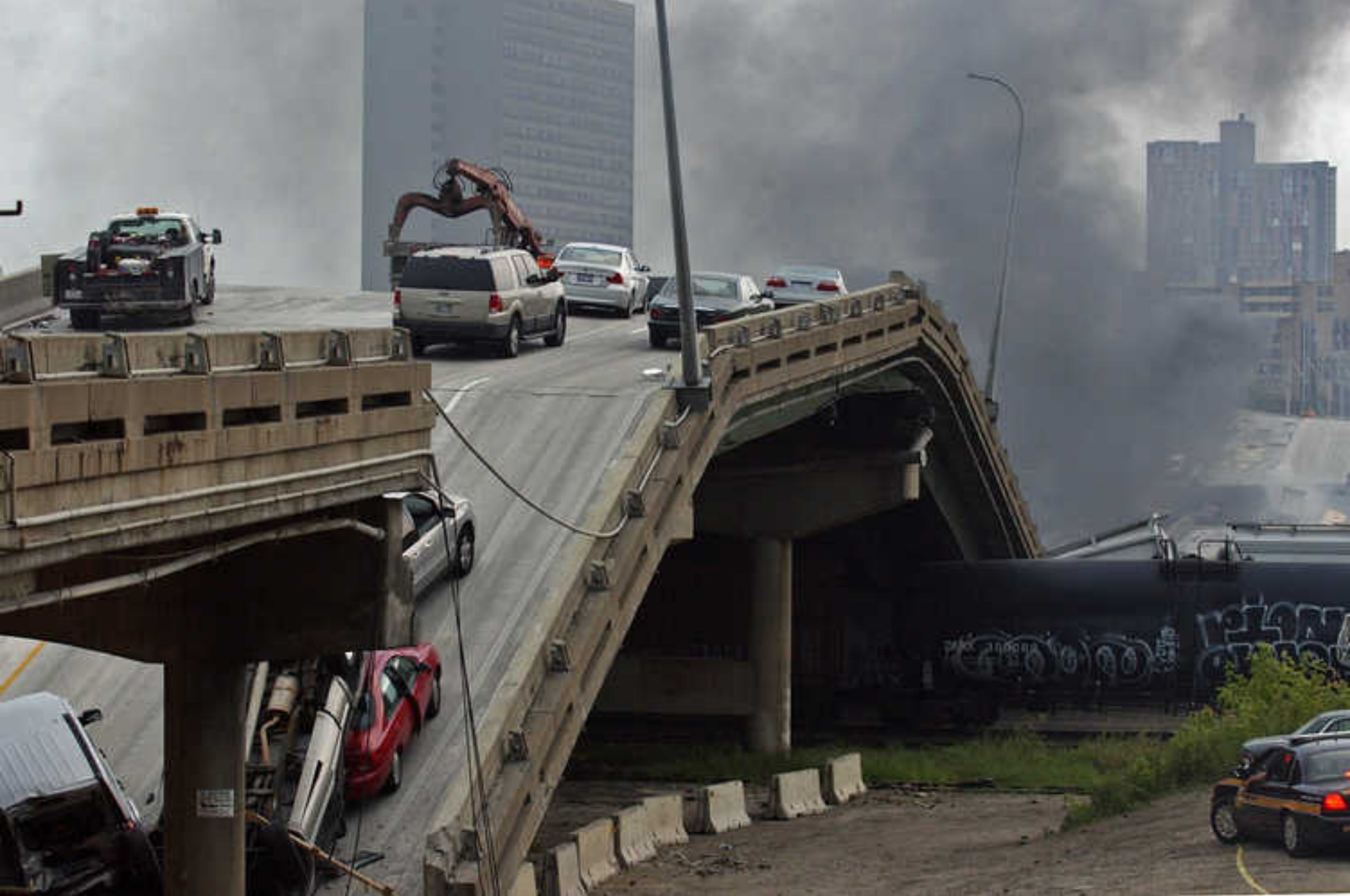
Presentation 05 - Photo of post-collapse vehicles
