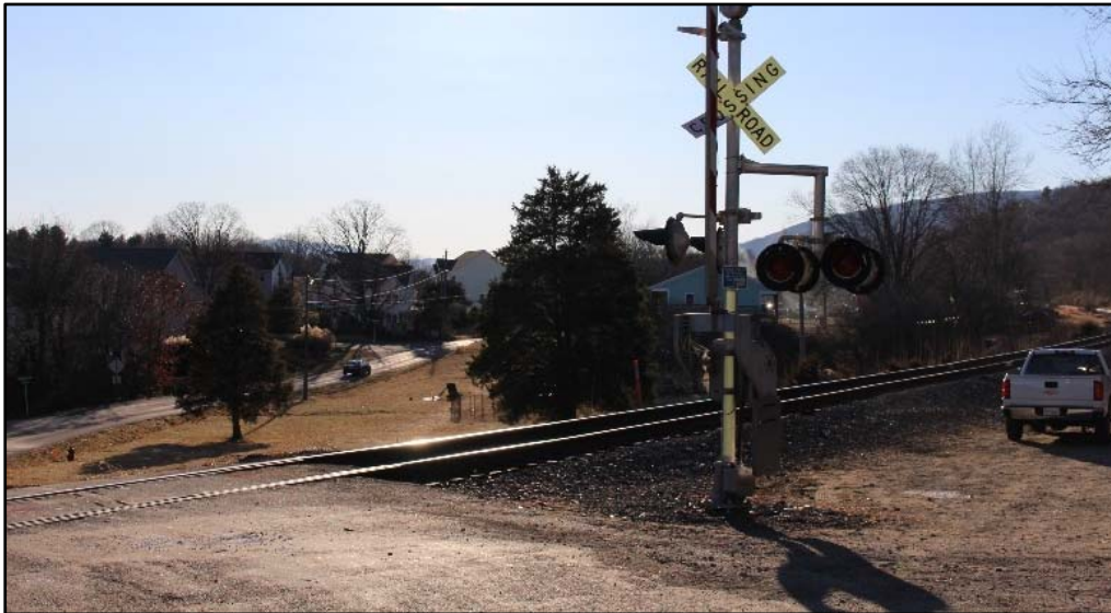
Figure 1. Southbound view of highway–rail grade crossing showing active warning devices.
