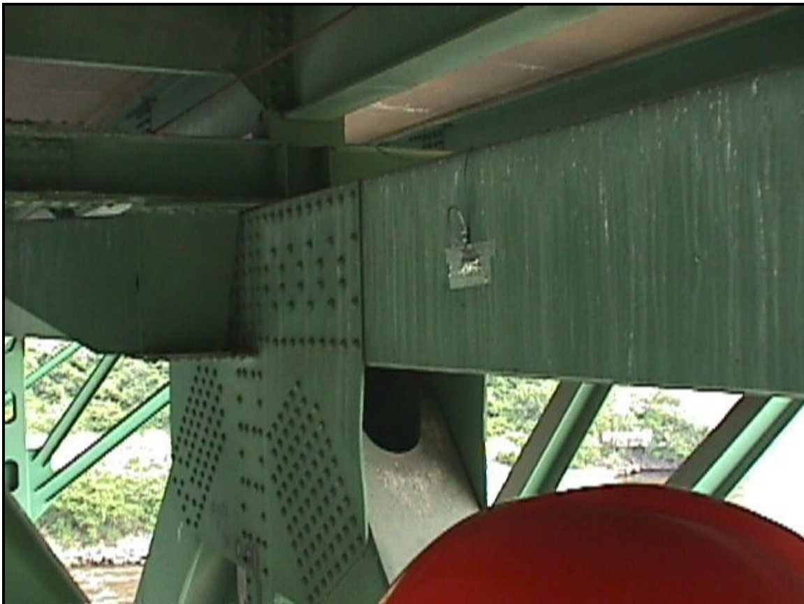
U10East , Source University of Minnesota (August 1999), MVC-010F.JPG
