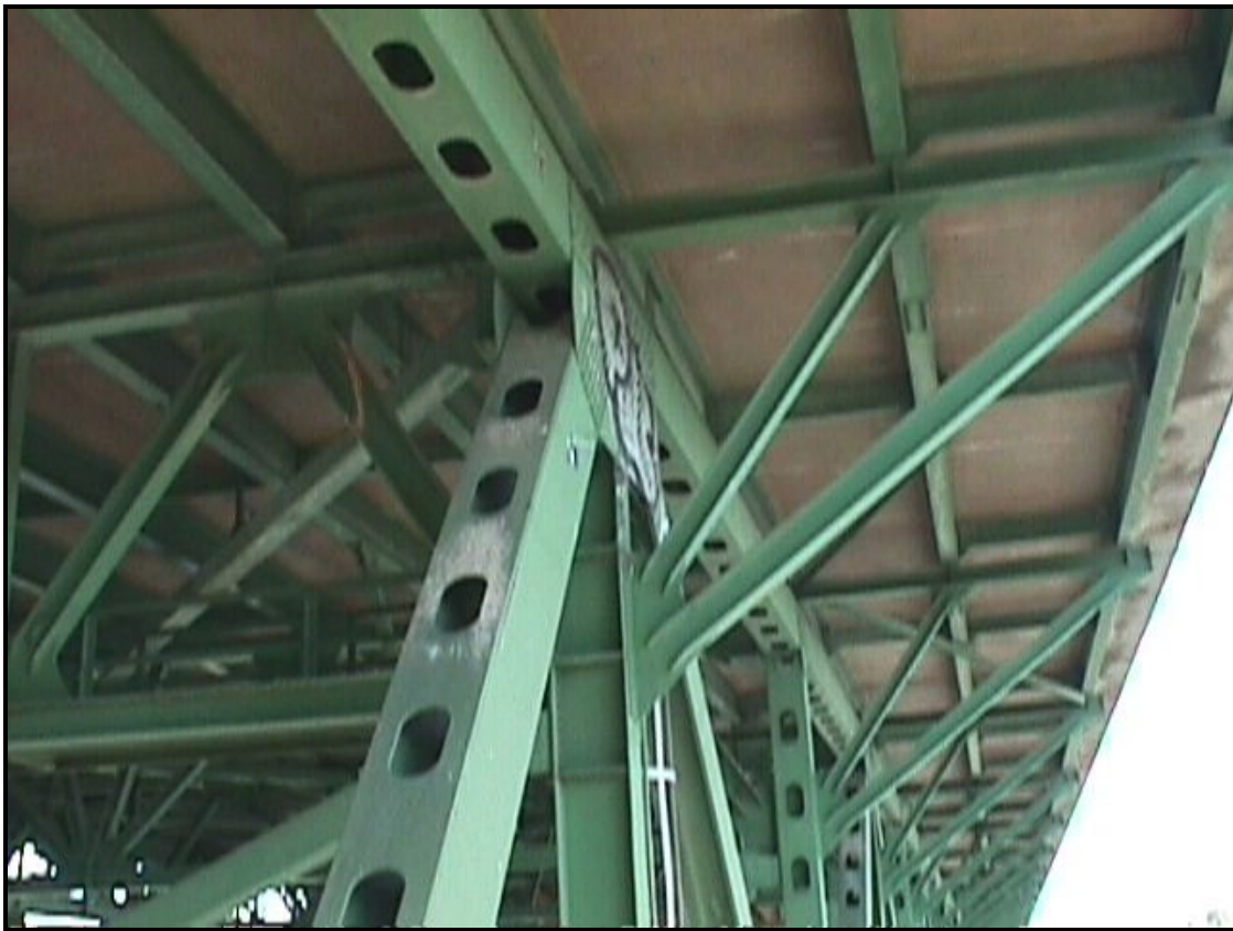
U10East , Source University of Minnesota (August 1999), MVC-011F.JPG
