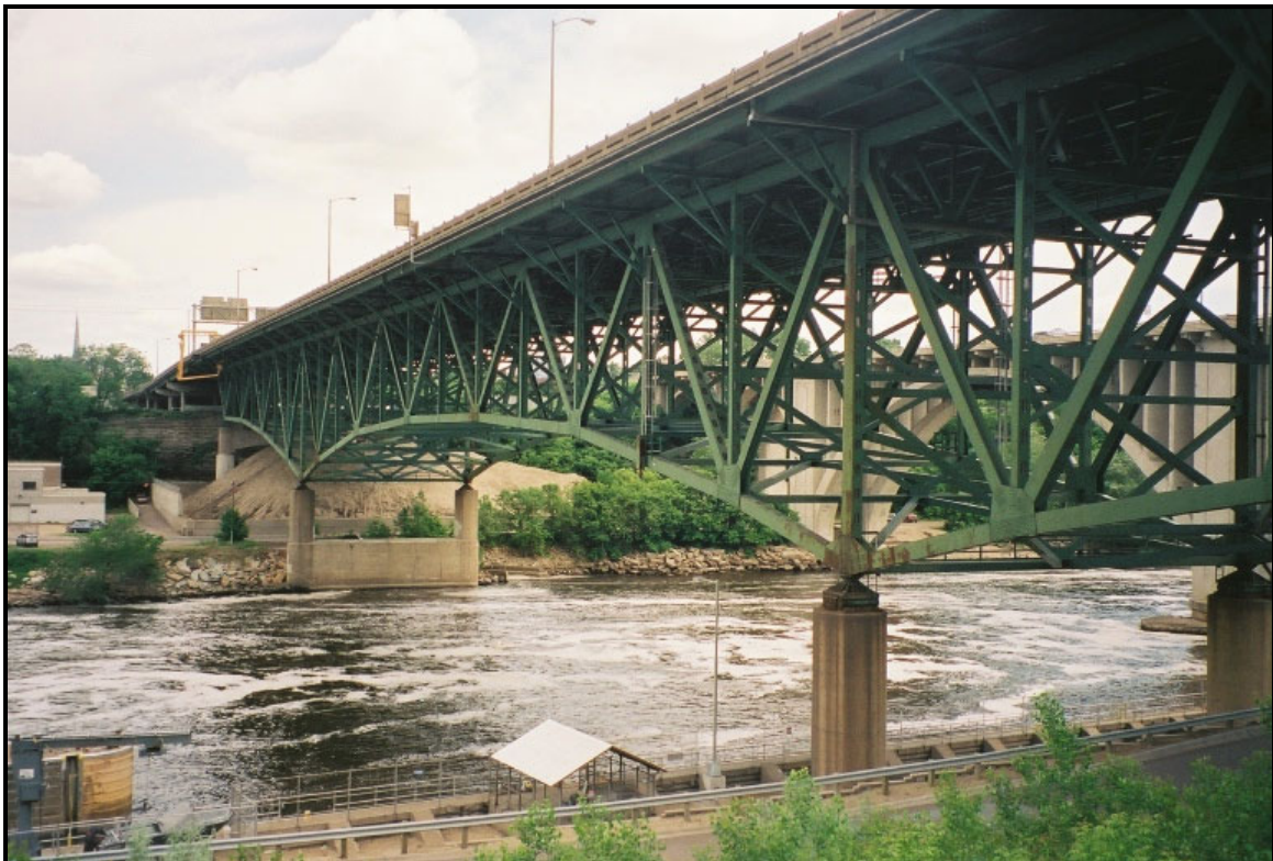
Overviews (West side of the Bridge), Source MNDOT Inspection 2003, D89426-R1-9.jpg
