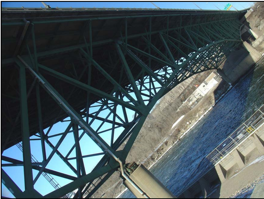
Overviews (East side of the Bridge), Source Individual, DSC07299.JPG
