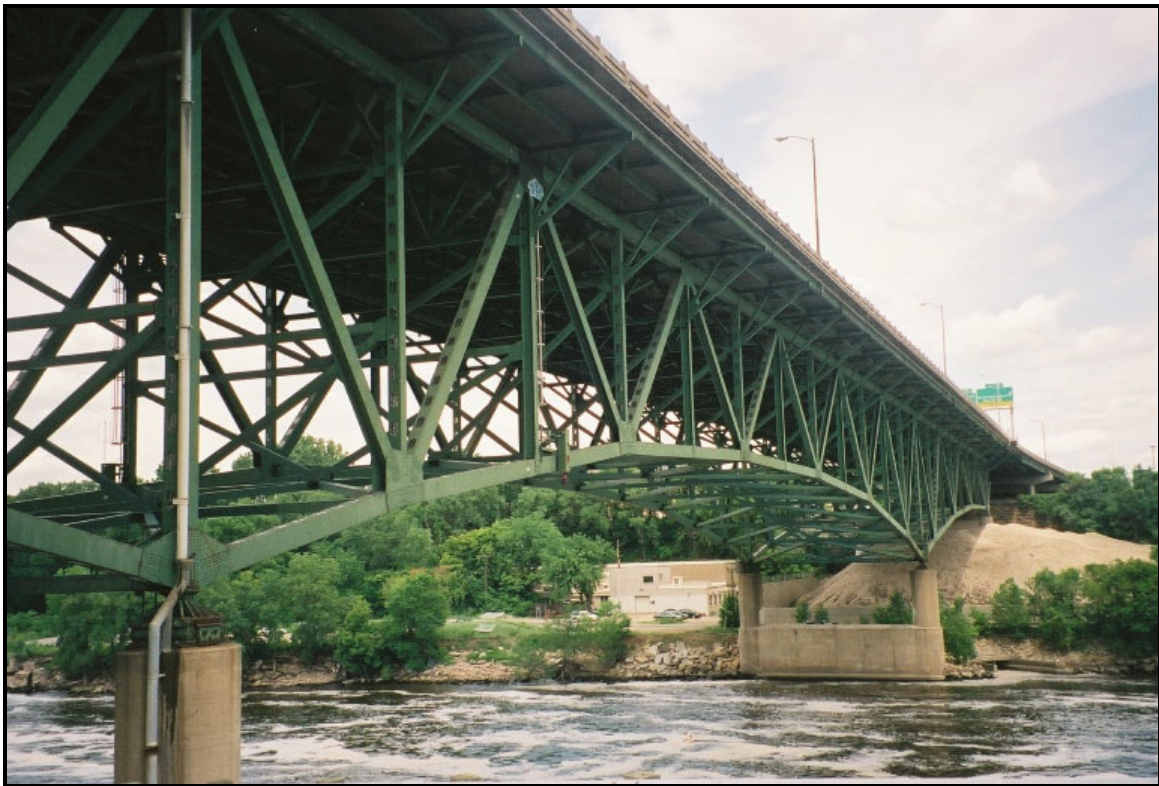
Overviews (East side of the Bridge), Source MNDOT Inspection 2003, D89426-R1-8.jpg
