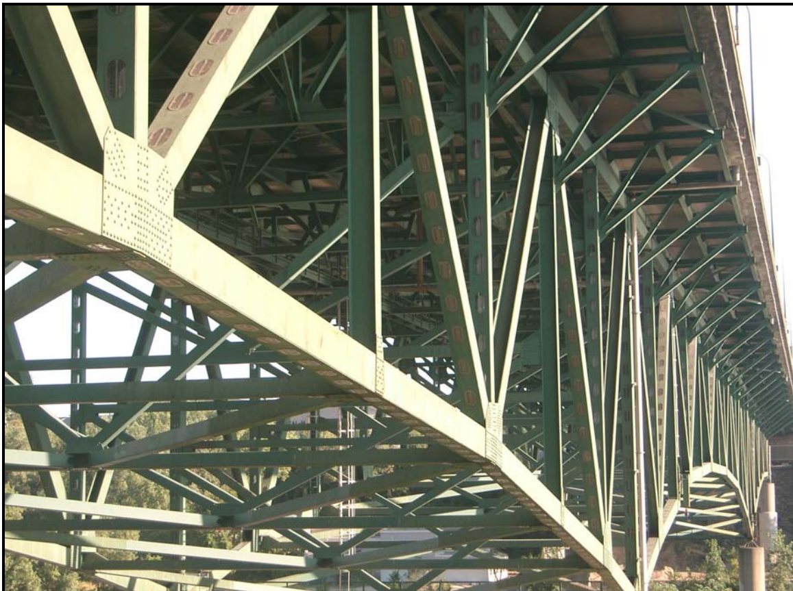
Overviews (East side of the Bridge) , Source Individual, CIMG8723.jpg
