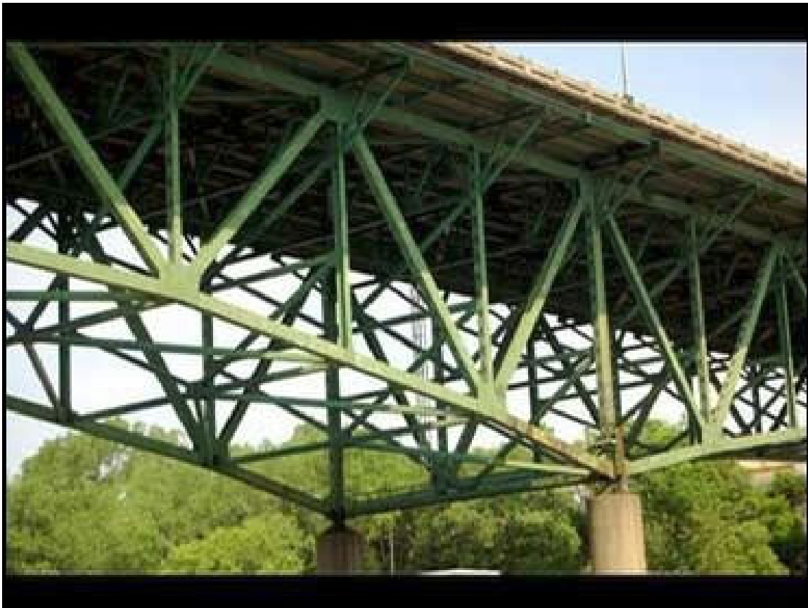
Overviews (East side of the Bridge) , Source University of Minnesota, 10.jpg
