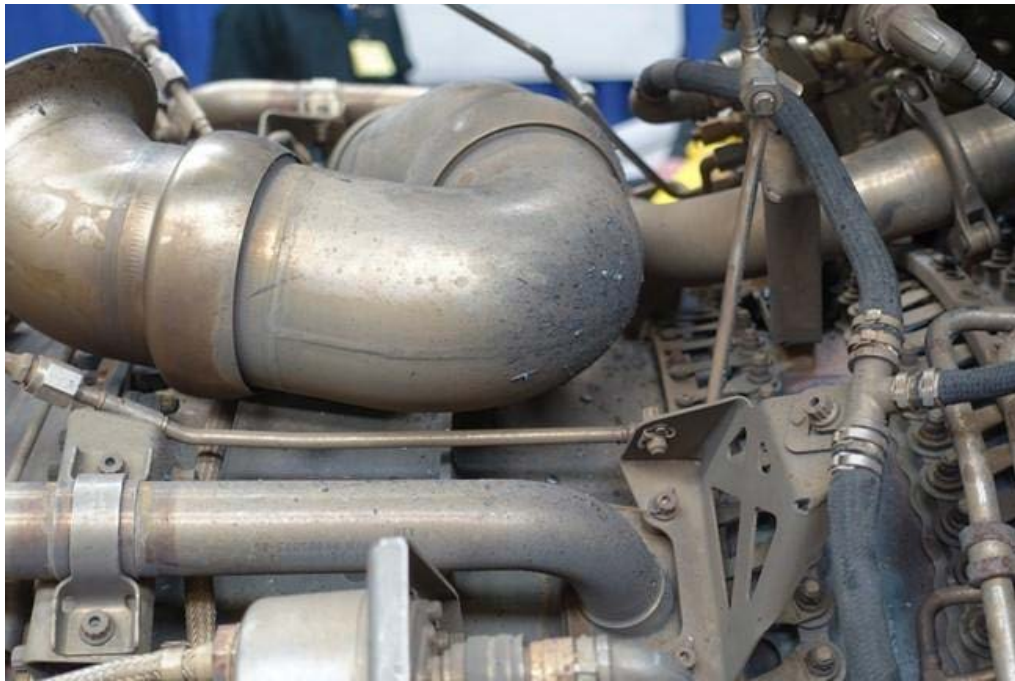
Photo 5- Metal Spray on Ducting Adjacent to Case Burn through (12 o'clock)
