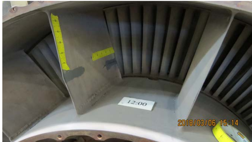
Photo No. 44: View of buckled turbine exhaust case strut. Also shown are the 9th stage turbine blades showing that they are all intact.(P&W)
