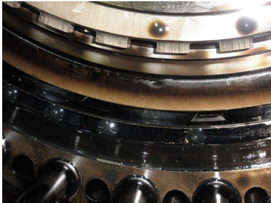
Photo No. 49: Close up of No. 1 bearing balls showing they are wet with oil and have no visible rotational distress.
