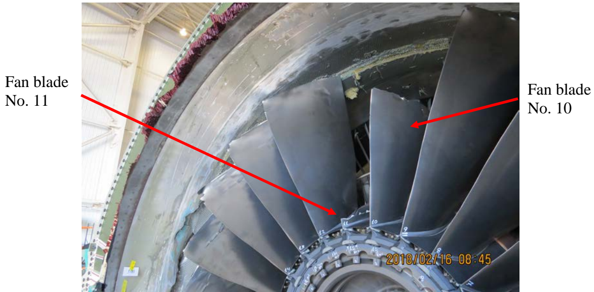
Photo No. 10: View of fractured fan blades Nos. 10 and 11. (P&W)
