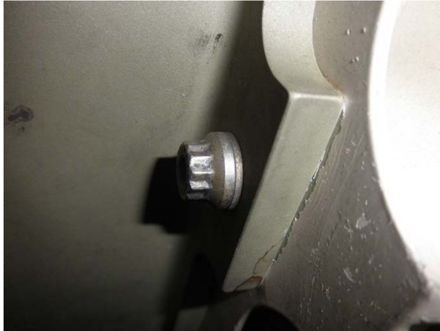
Photo No. 15: Close up of rear face of inlet duct showing paint scraped up adjacent to the engine's fan case front flange.
