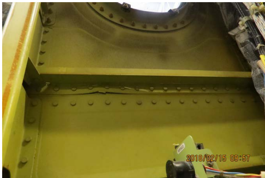
Photo No. 59: View of underside of bent and cracked zee stringer at BSTA 913. (P&W)
