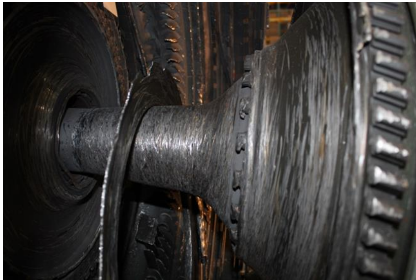
Photo 15- LPT Shaft and LPT 6 th Stage Disk Hub Scoring Damage
