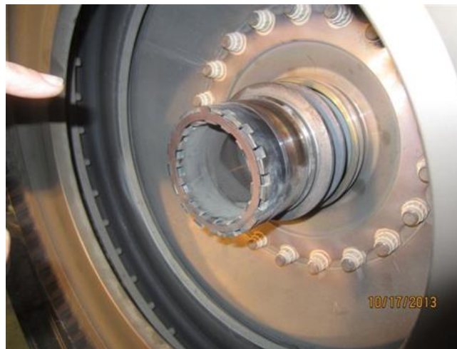
Photo 16- No. 5 Bearing, Rollers and Outer Race Missing. No. 5 Bearing Lock Ring and Nut Intact
