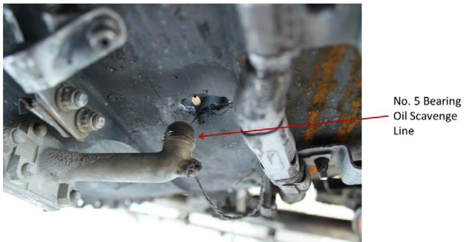
Photo 9- No. 5 Bearing Oil Scavenge Line
