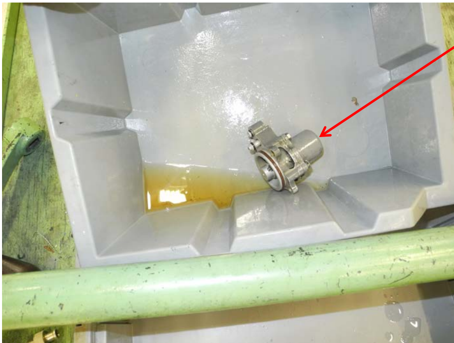
Figure 20 – Fuel Drained from Filter Cavity
