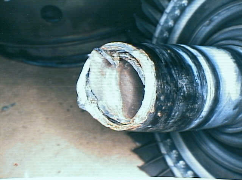
Powerplants 8 - Photo 36. Left engine combustion chamber liner
