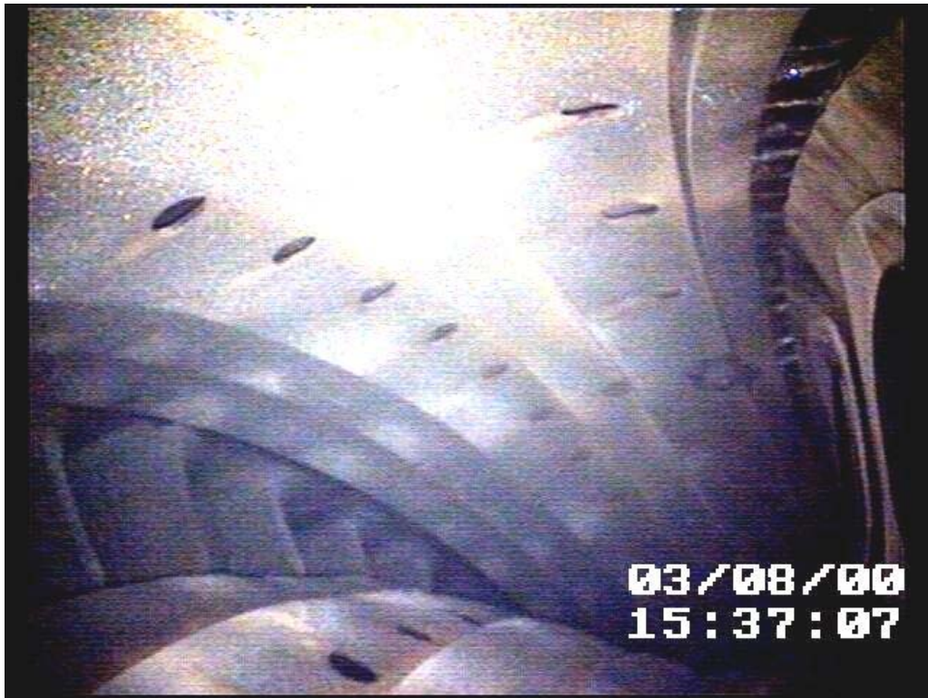
Photo 5: No. 1 engine combustion chamber
