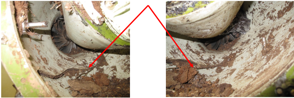
PHOTO 3: LOWER LEFT-HAND LOOKING THROUGH INLET
