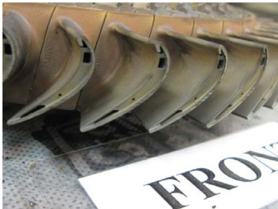
PHOTO 20: 1 ST -STG TURBINE ROTOR BLADE TIP SCORING
