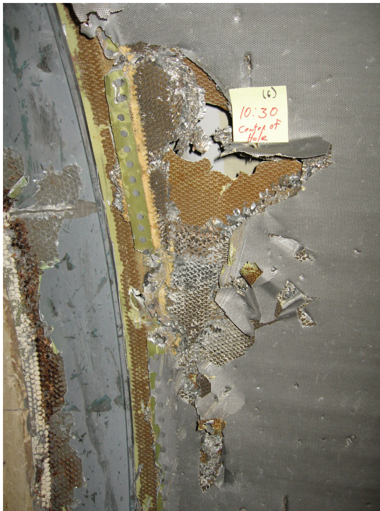
PHOTO 9: INLET COWL INNER BARREL DAMAGE - LOCATIONS 3 AND 4
