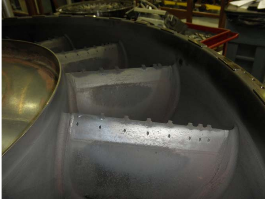
Photo No. 19: Close-up view of the turbine exhaust case inner and outer ducts and struts showing dark discoloration all around and the elliptical-shaped areas on the struts.
