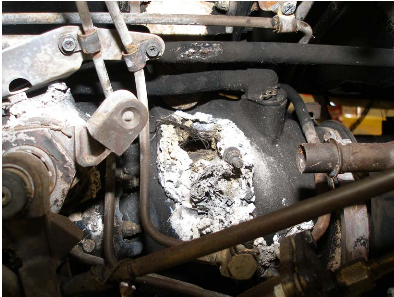
Photo No: PA290043.tif
