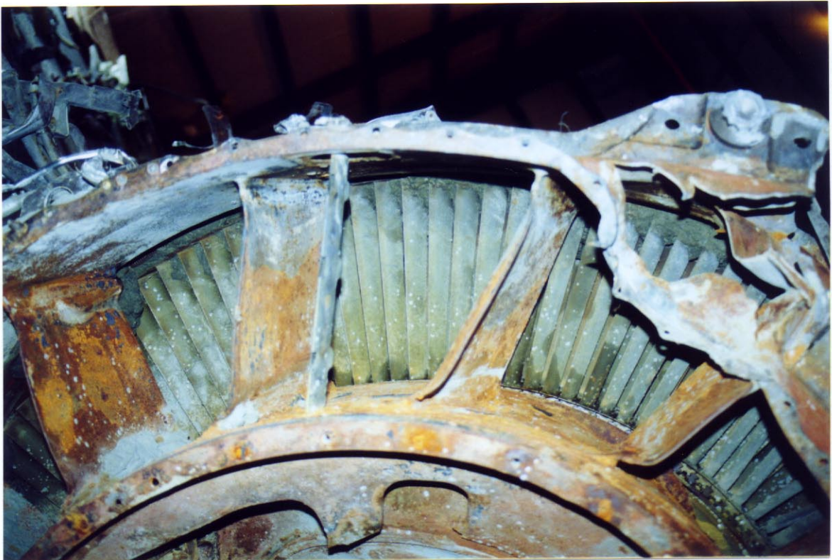
Photo 7. Closeup of rear of No. 1 engine showing full length 6 th stage turbine blades.
