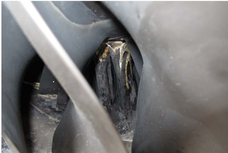
Photo 4- Fan Stator as Viewed Through the Fan (6 o'clock)
