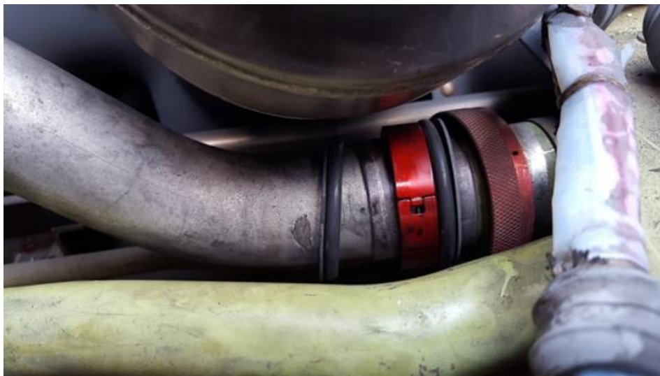
Photo 11- Fuel Coupling Assembly, As Found In-situ
