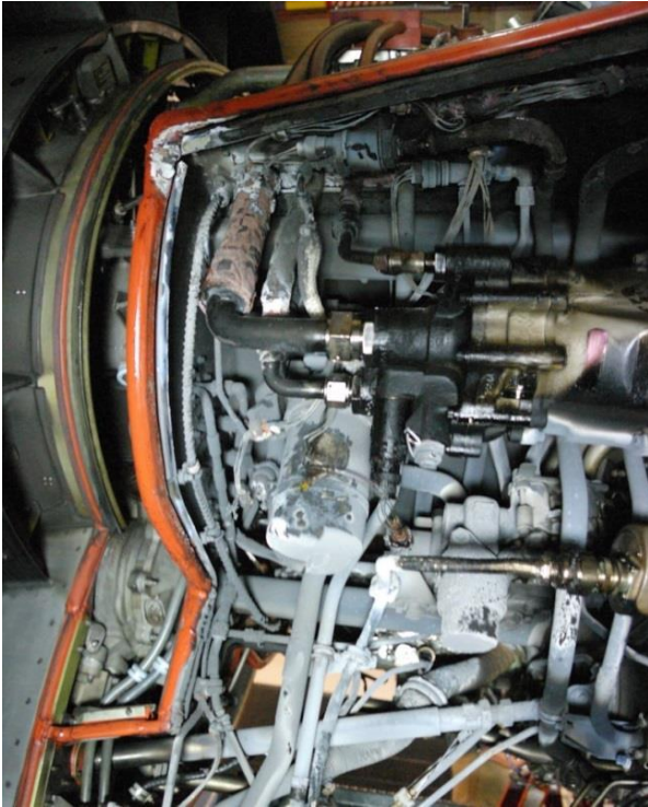
PHOTO 8: FIRE DAMAGE ON LEFT SIDE OF ENGINE UNDERNEATH HEATSHIELD
