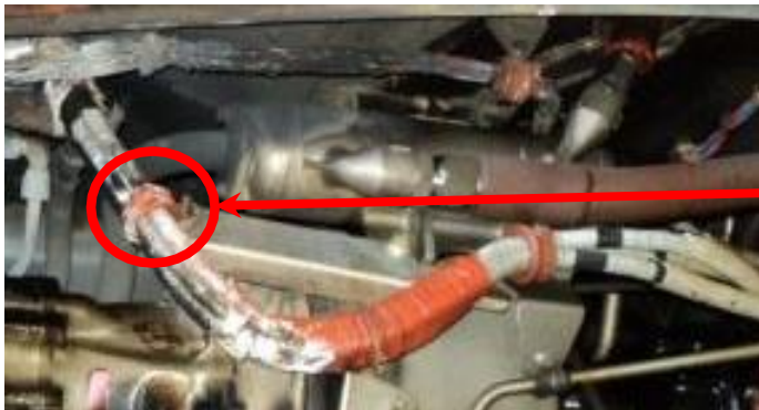
PHOTO 30: EVENT ENGINE IDG POWER FEEDER CABLE ORIENTATION WITH FORWARD P-CLAMP DOWN
