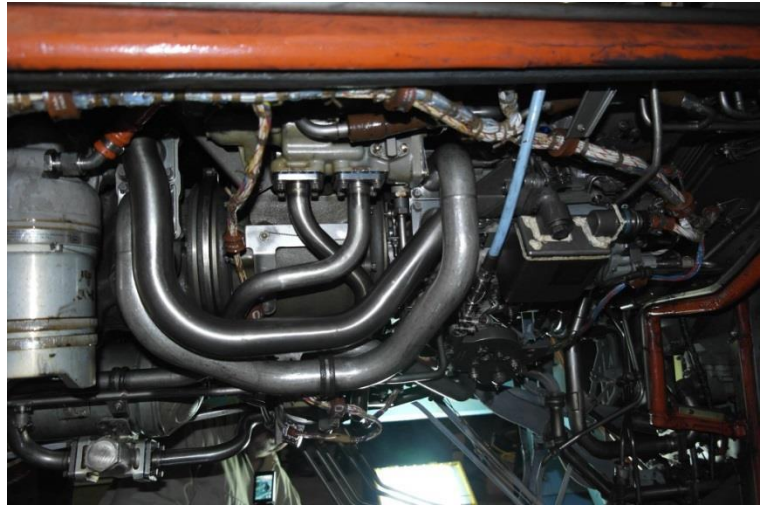
PHOTO 9: NO FIRE DAMAGE ON RIGHT SIDE OF ENGINE UNDERNEATH ENGINE HEATSHIELD
