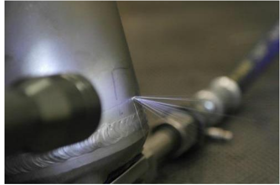
PHOTO 19: LEAK AT 60 PSI FLUID PRESSURE
