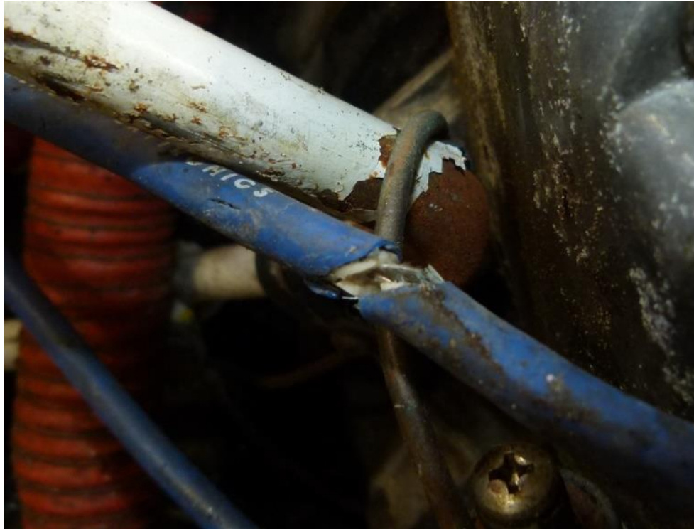
Figure 9 - Exemplar Ignition Lead Cut
