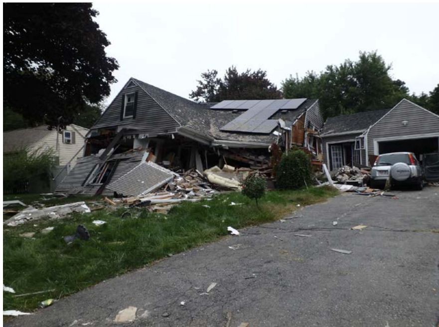
Figure 1-- Damaged home where fatality occurred
