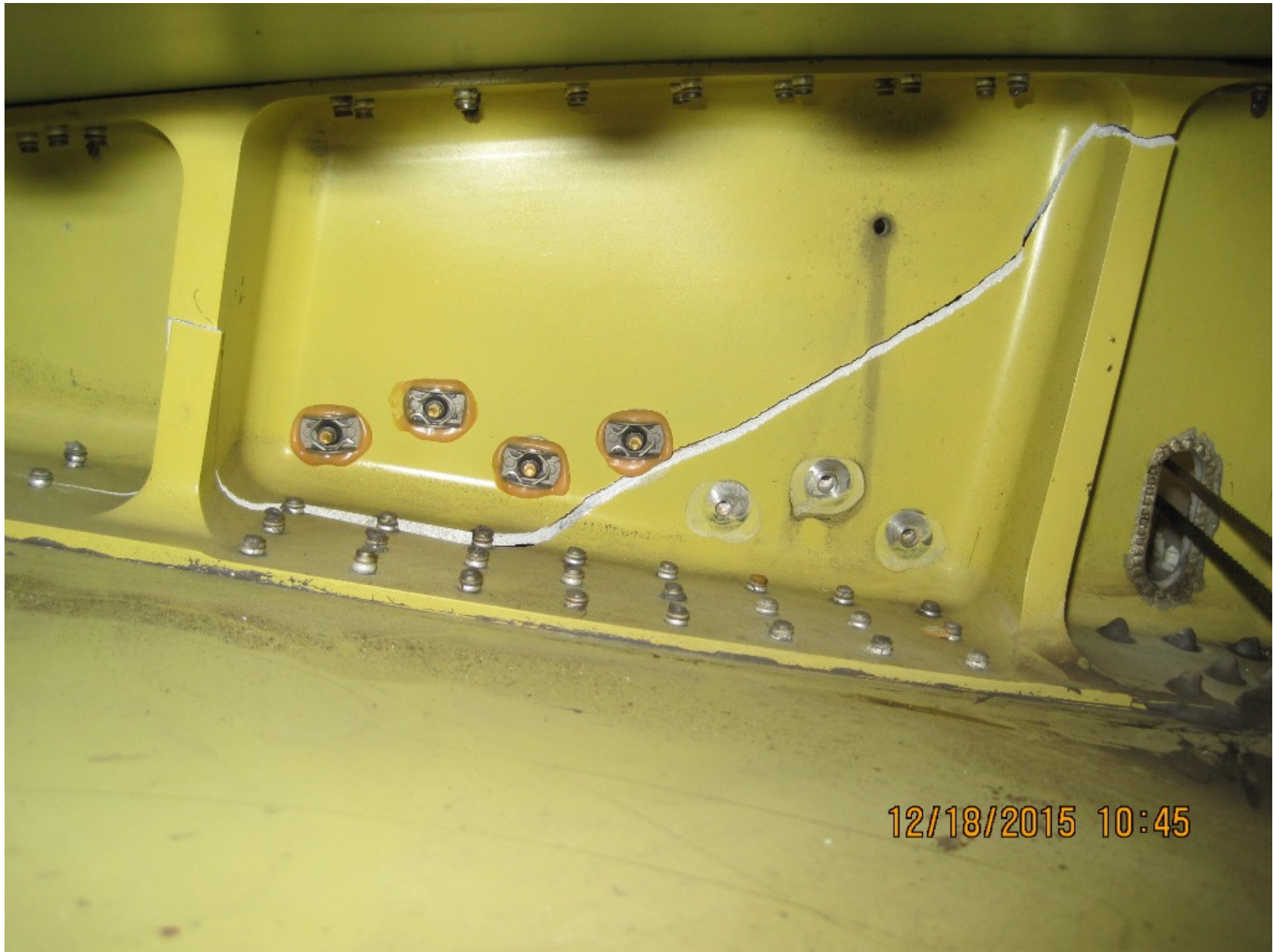
Photo 3 – View of damage to right wing rib (Courtesy of FAA)
