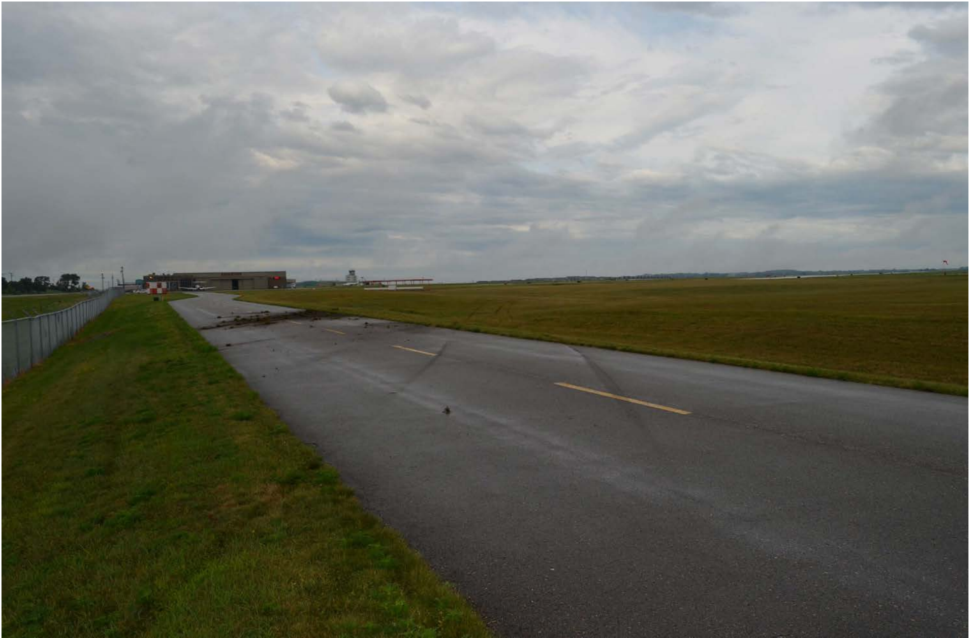
Photo 3 - Photo taken at 0901 – View of airport perimeter road looking southwest
