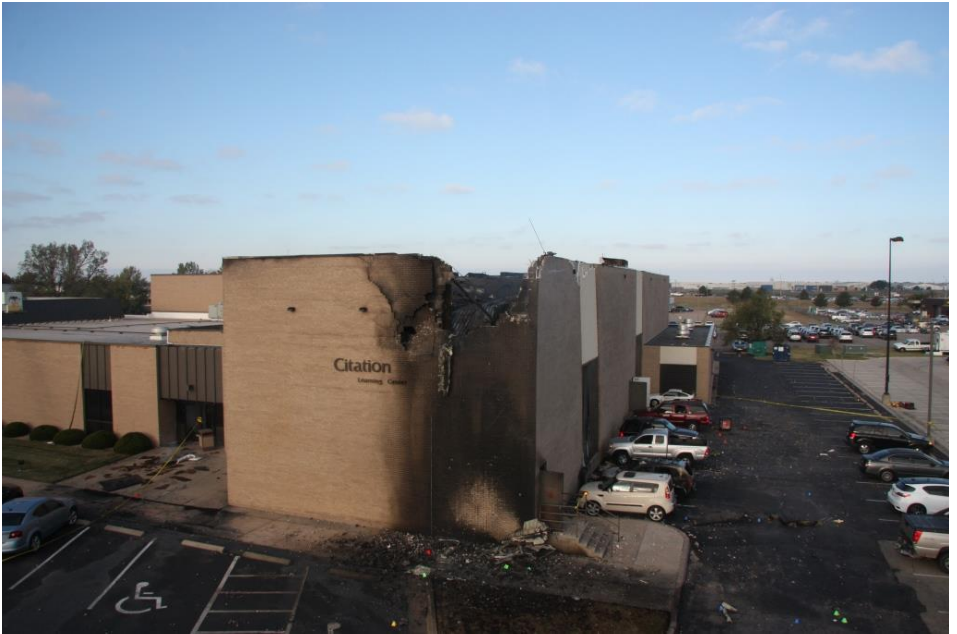
Photo 4 – Aerial view of impact point
