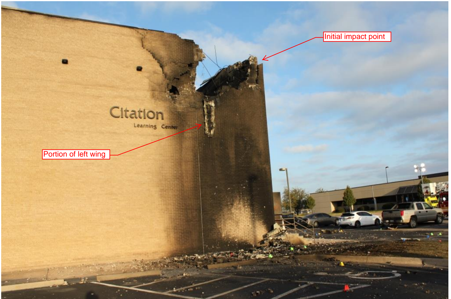
Photo 1 – Initial Building Impact
