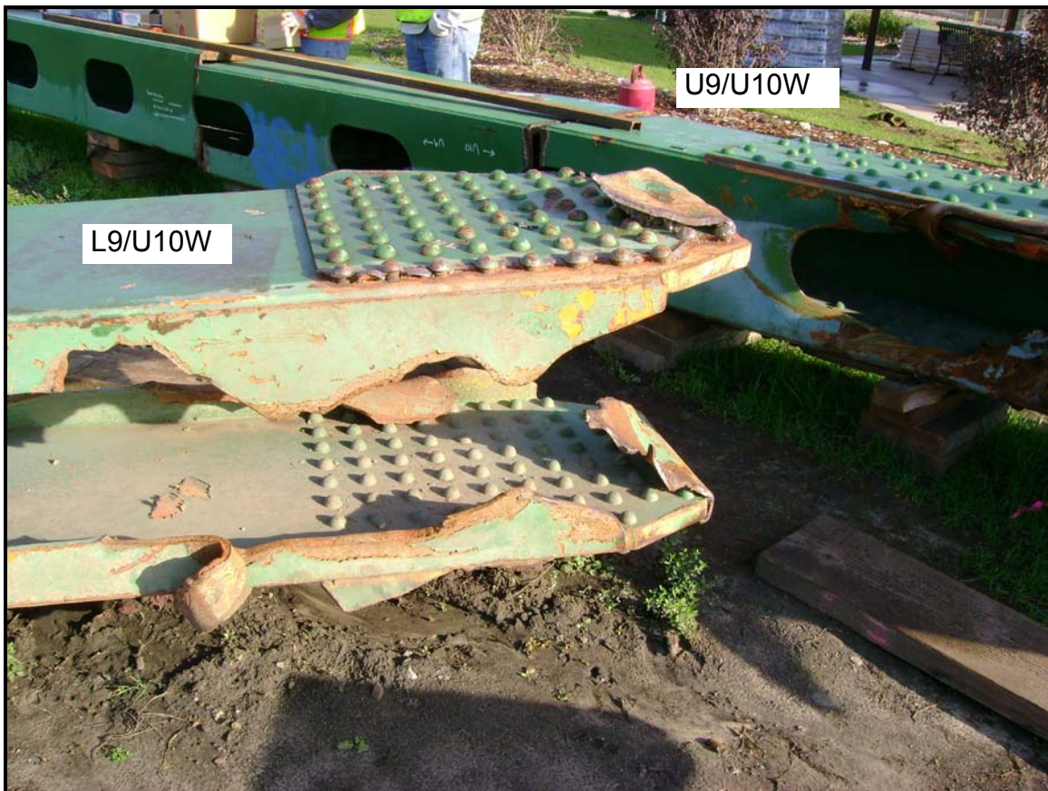
Node U10 West, showing L9/U10W in foreground and U9/U10W in background.
