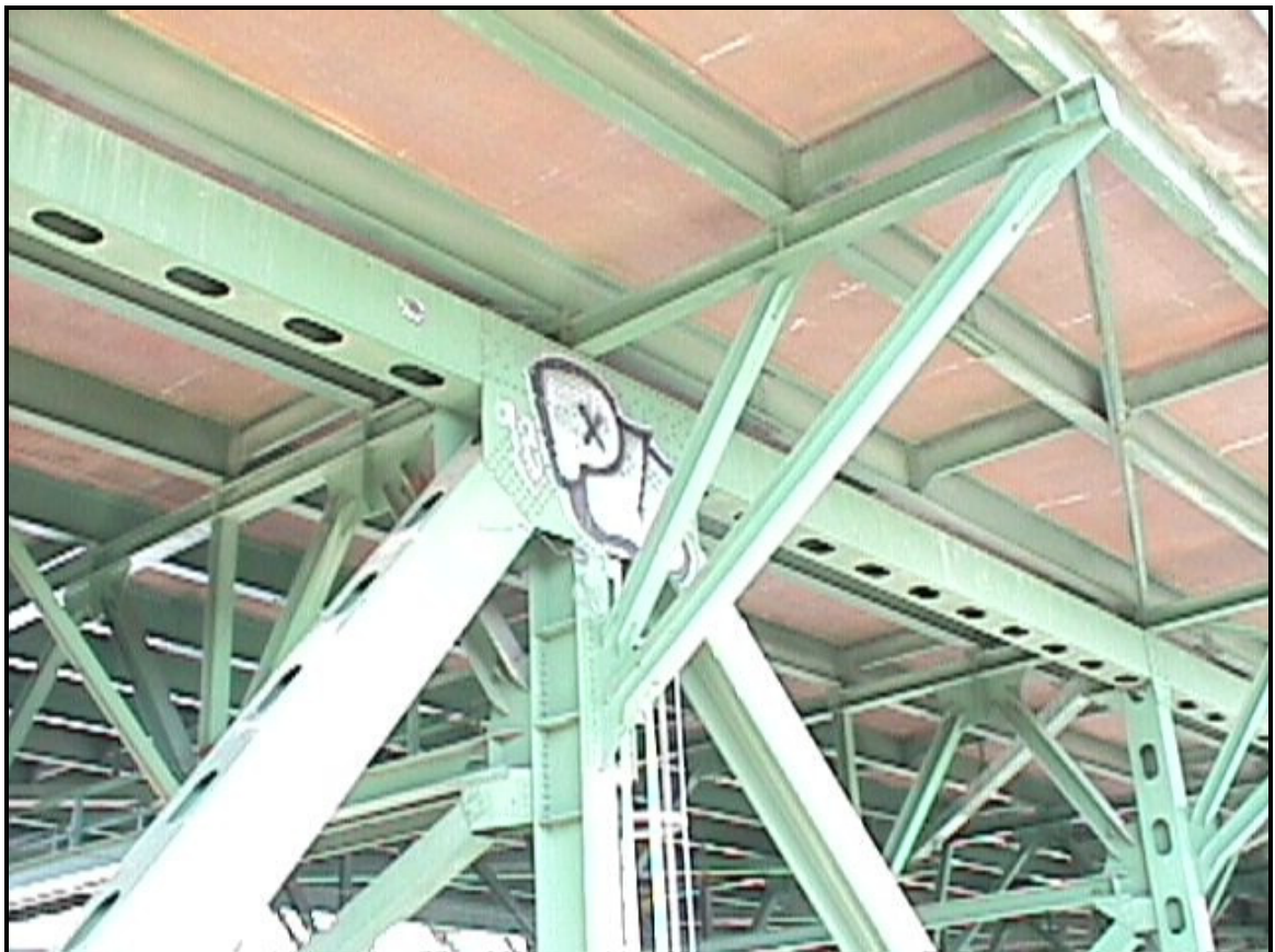
Looking northwest at node U10 East of the deck truss.
