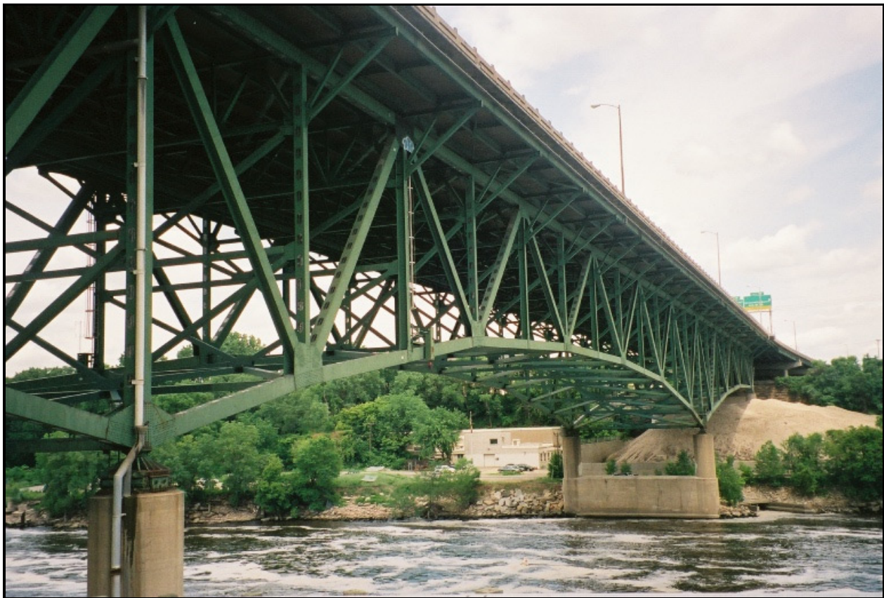
A view of the east side of the deck truss portion of the bridge, looking northwest.
