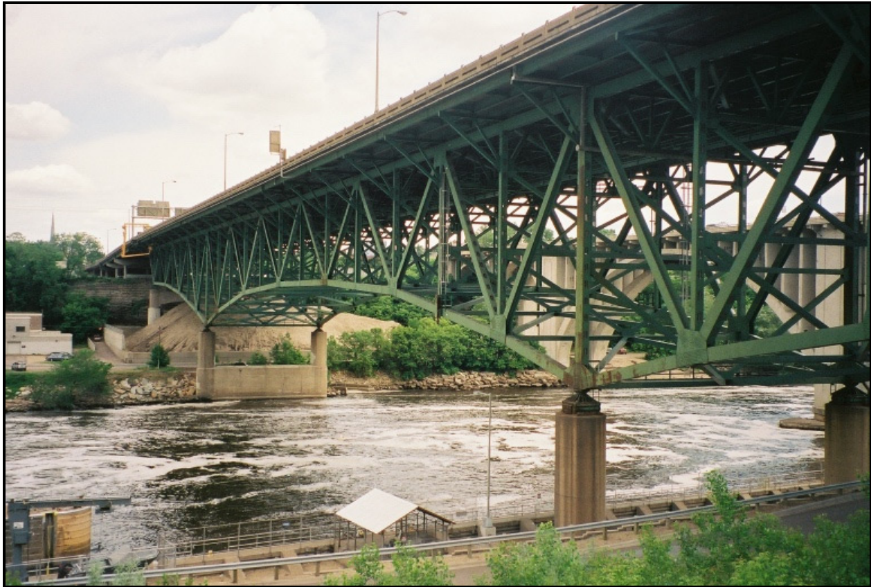
A view of the west side of the deck truss portion of the bridge, looking northeast.
