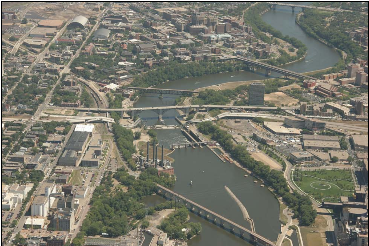
Post collapse view of the bridge and surrounding area, viewed looking east.
