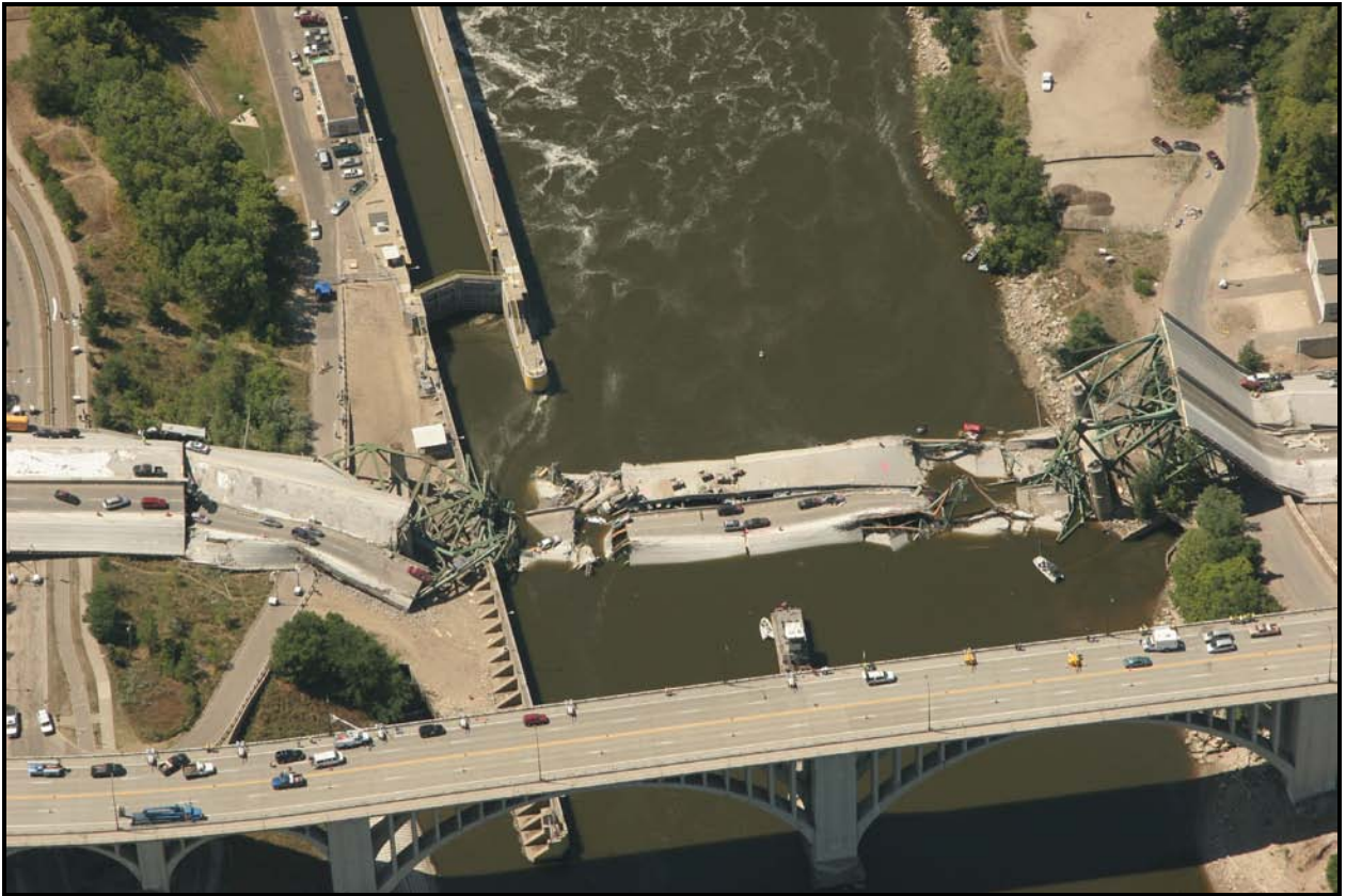
Post collapse, viewed looking west.
