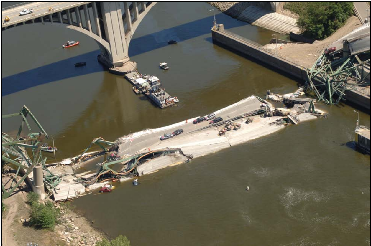
Collapsed portion of the deck truss over the river, viewed looking east and south.
