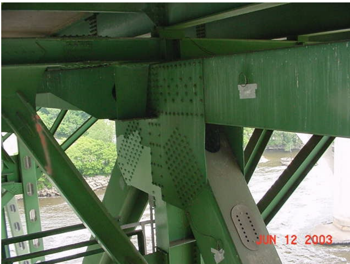
Node U10 East, viewed looking northeast from inside the structure.
