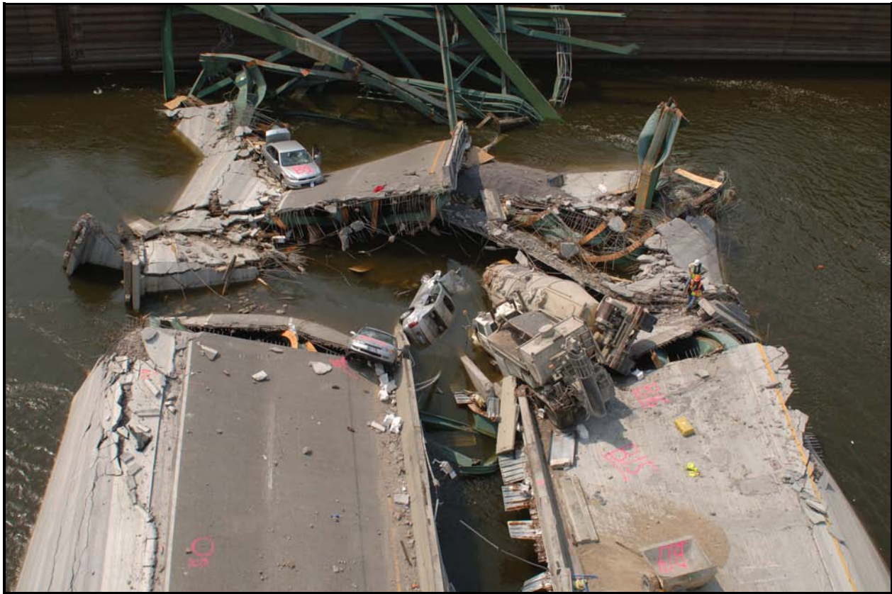
South portion of the center span, viewed looking south.
