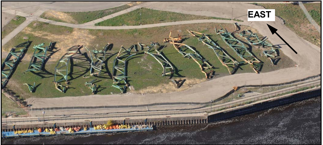
Bohemian Flats Layout showing the floor trusses, with the east ends of the floor trusses closer to the top of the photograph.
