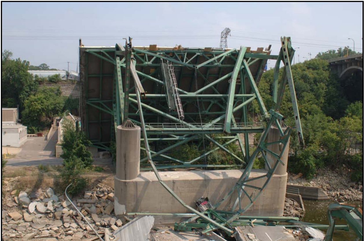
Damaged portion of the deck truss at pier 7, on the north side of the river, viewed looking north.
