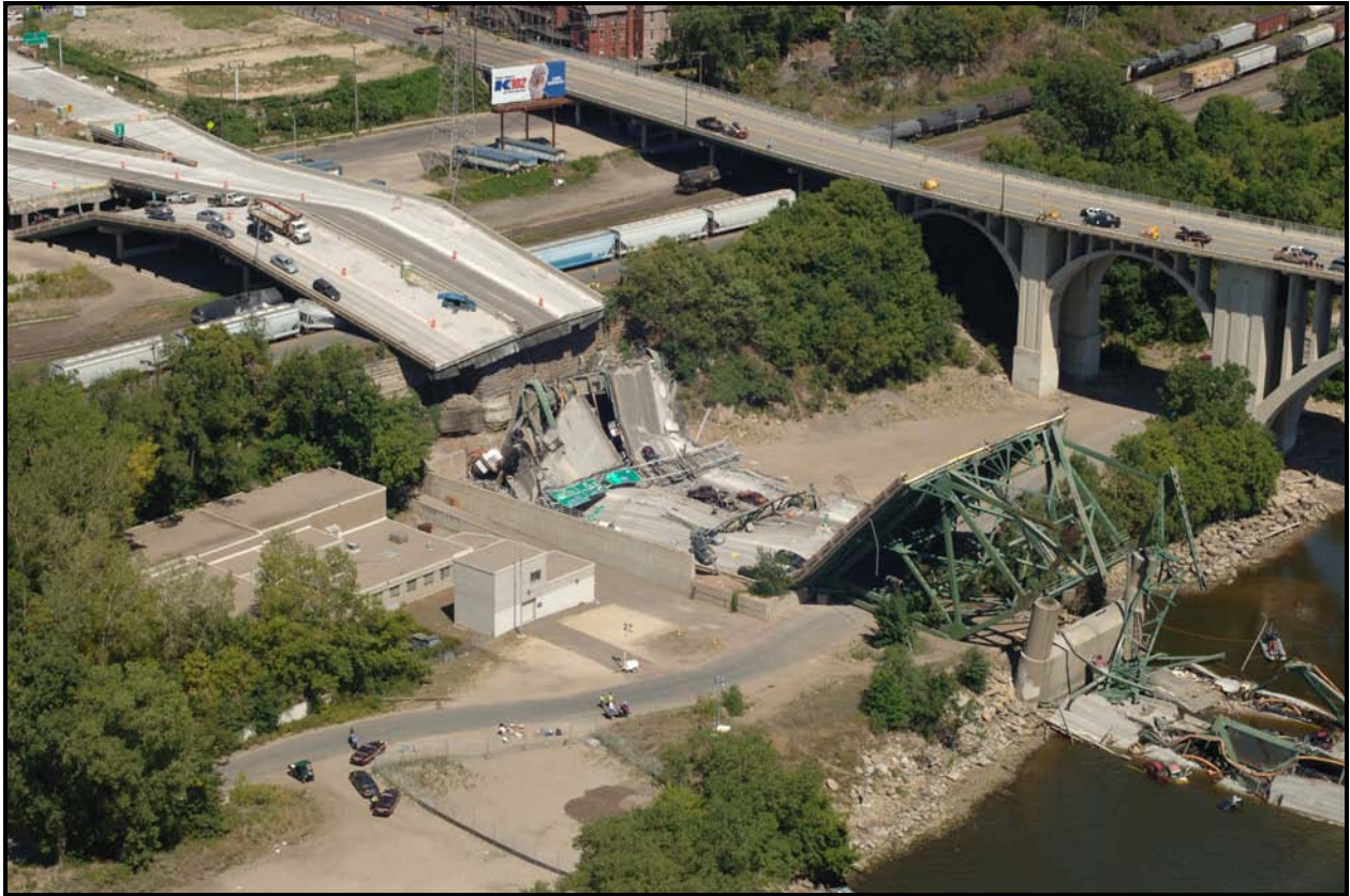
North portion of the collapsed bridge, viewed looking north and east.
