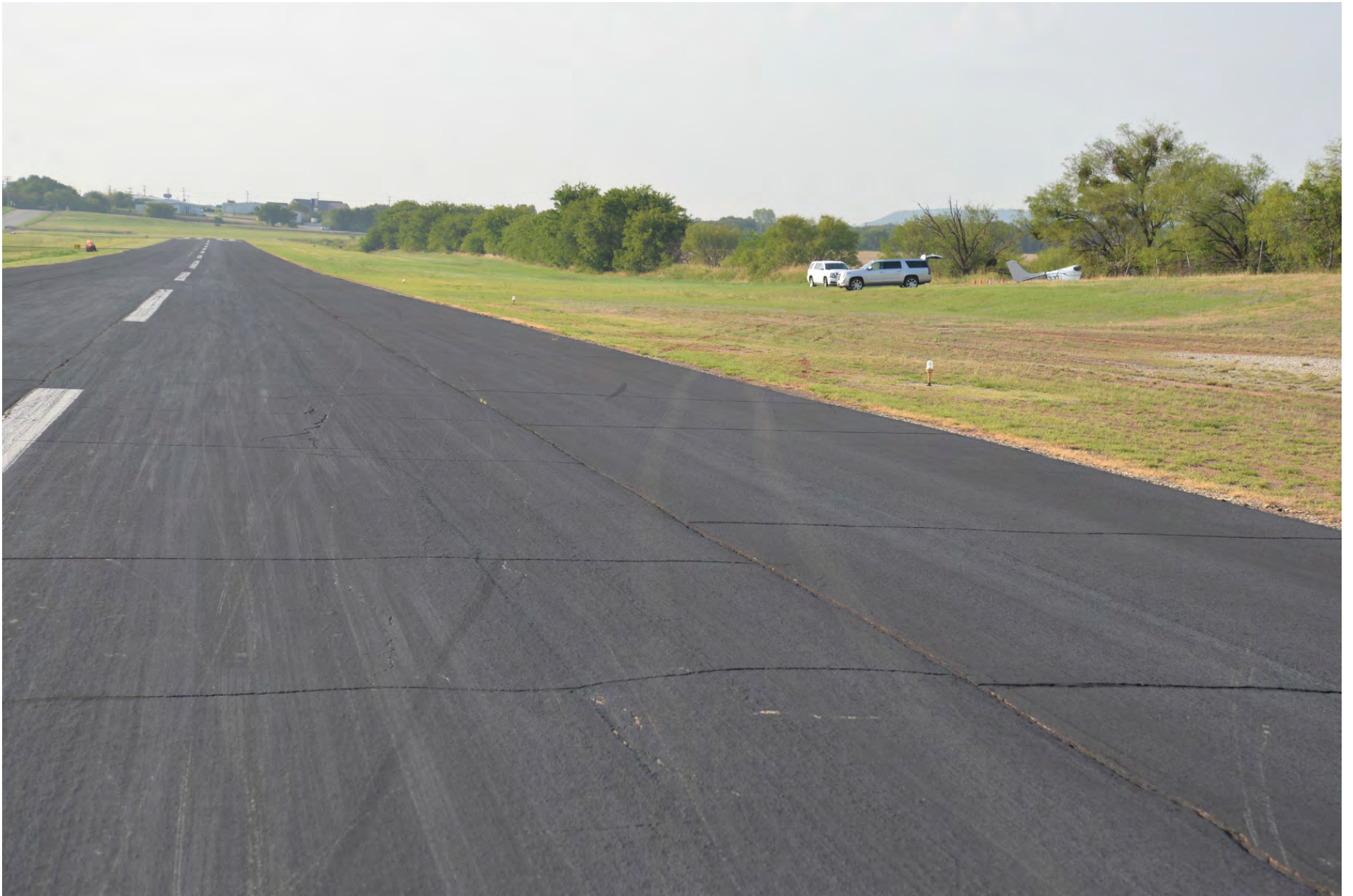
Photo 7 - Close-up view of the runway looking towards the wreckage.
