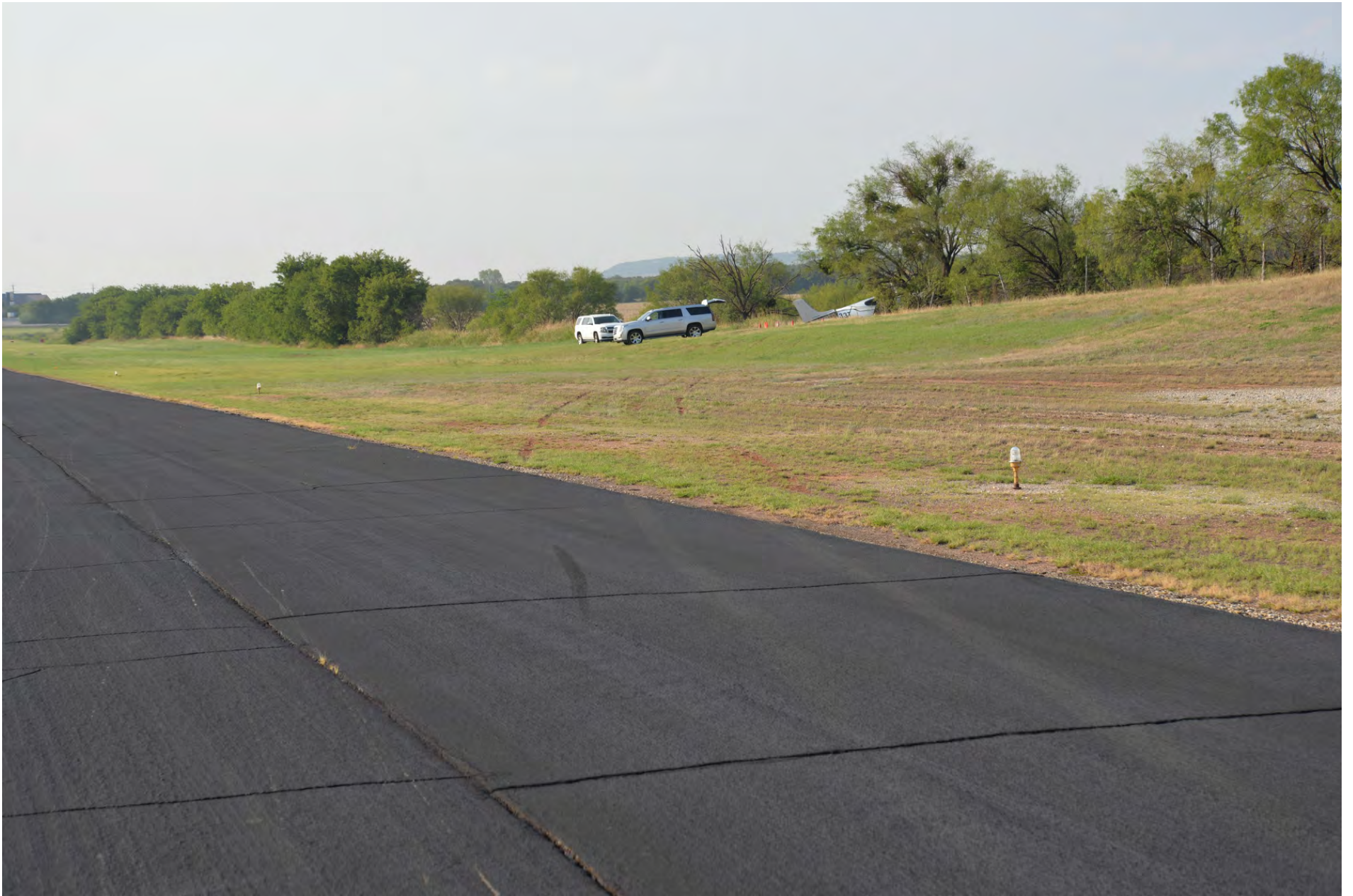
Photo 8 - Close-up view of the runway looking towards the wreckage.
