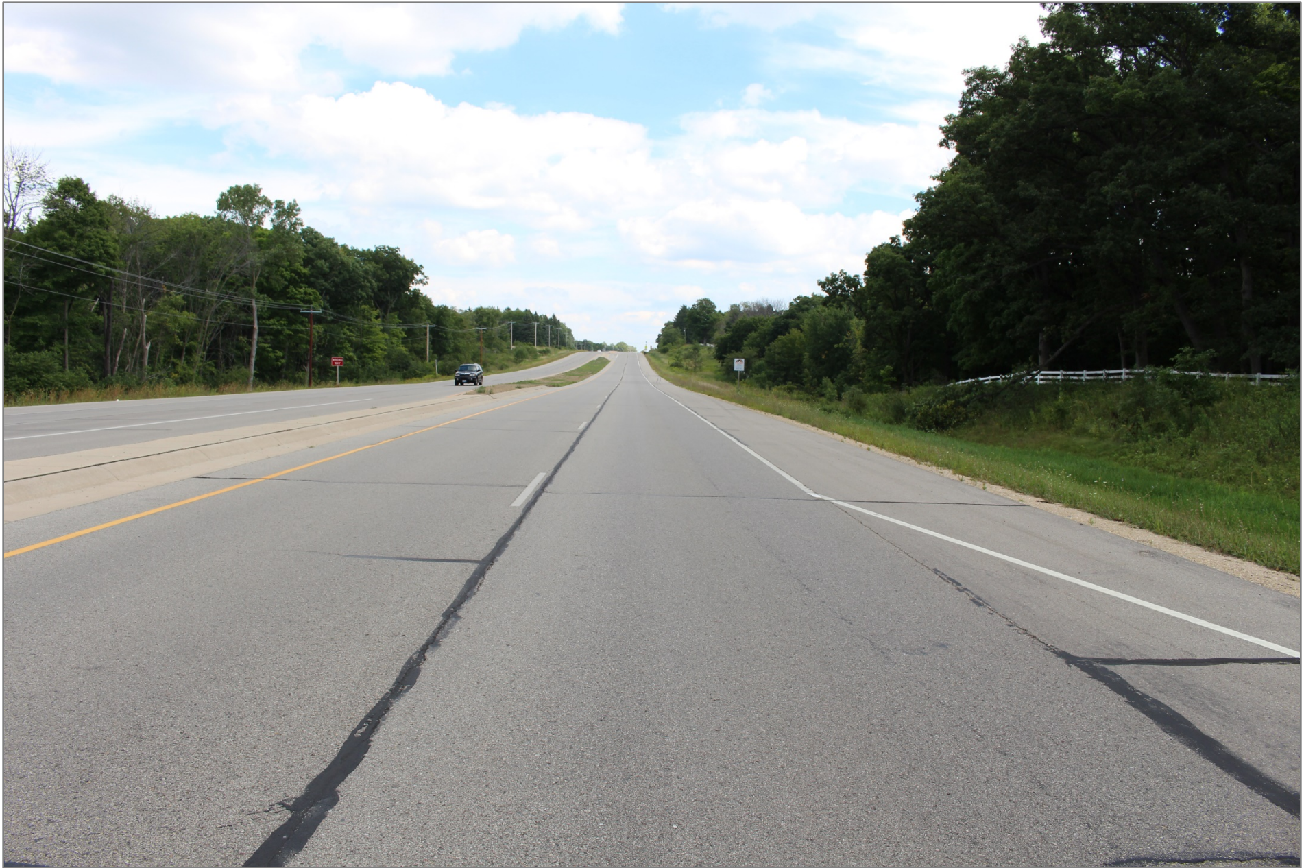
Photograph 1 – Eastbound Traffic Lanes at Crash Location – Facing East During Daylight Hours
