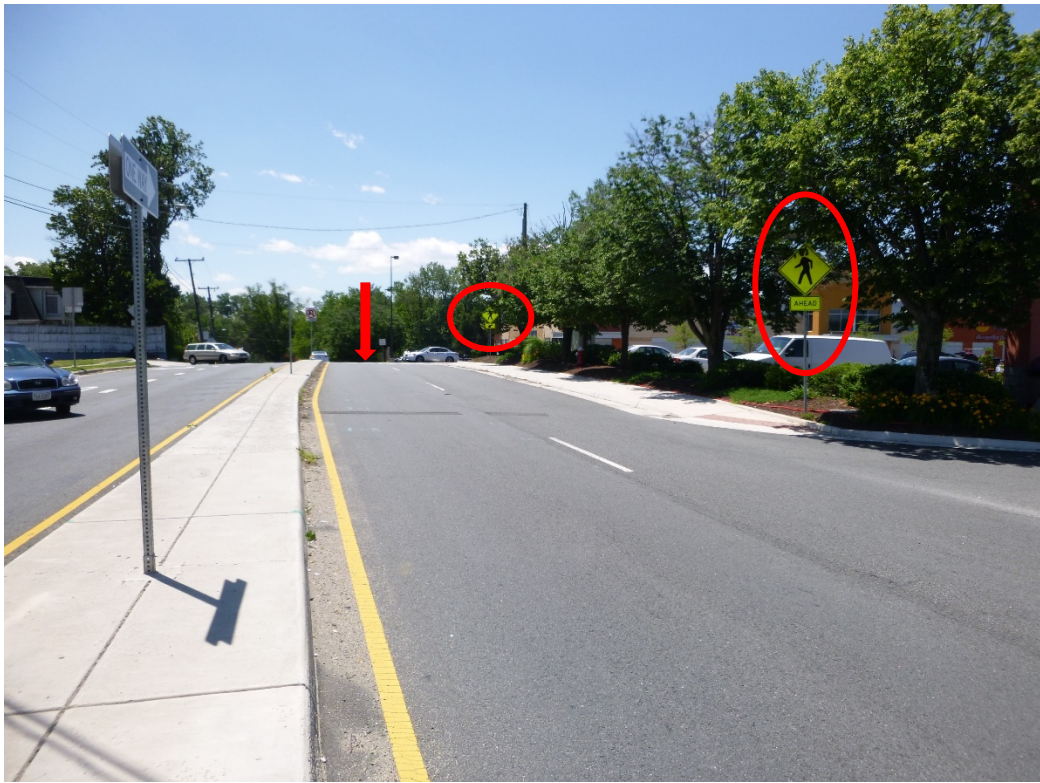
Photo 3 – A view facing southbound on Graham Road showing the crosswalk ahead plaque and the pedestrian warning signs with diagonal arrow plaque (circled in red) the area of impact is shown by the red arrow
